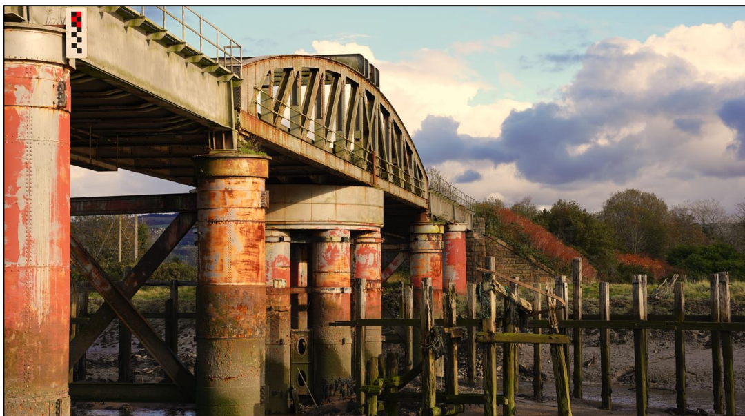
Figure 1: Neath Swing Bridge (taken from western shore).
