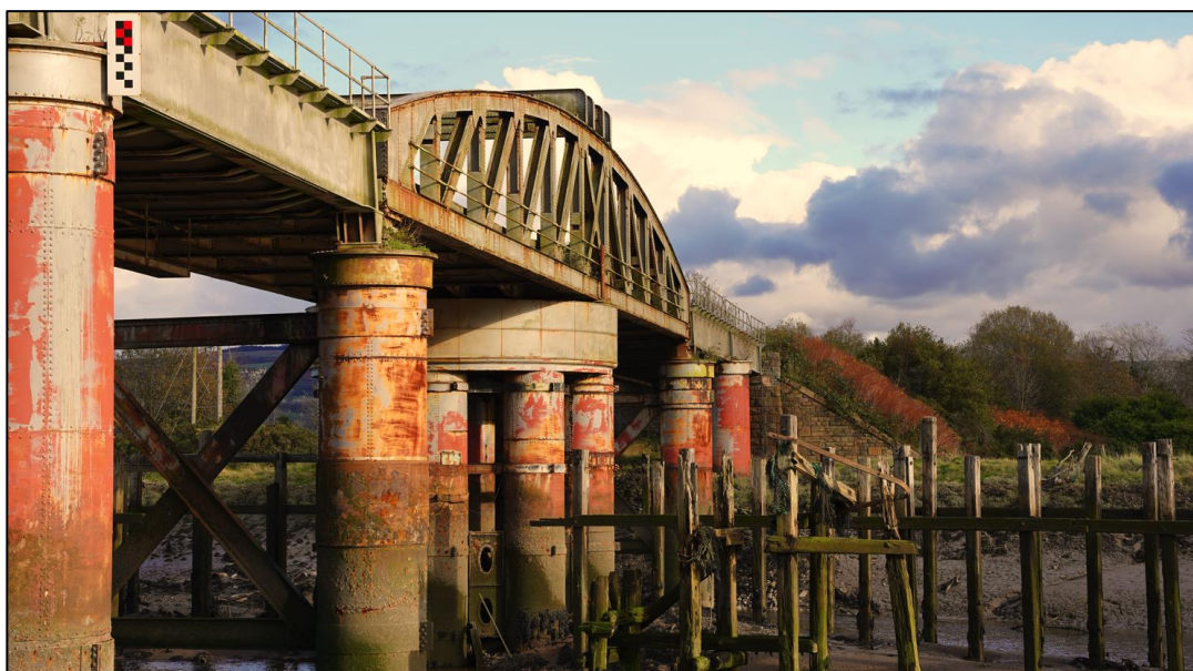
Figure 1: Neath Swing Bridge (taken from western shore).
