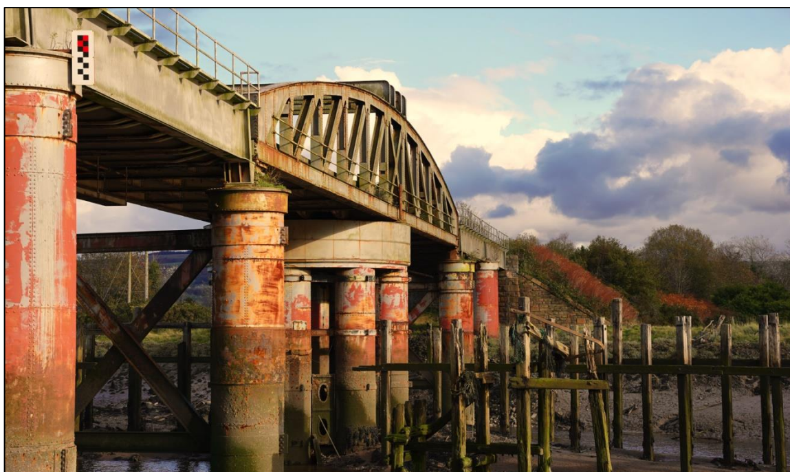
Figure 2: River Neath Swing Bridge from Western Shore (Facing East).
