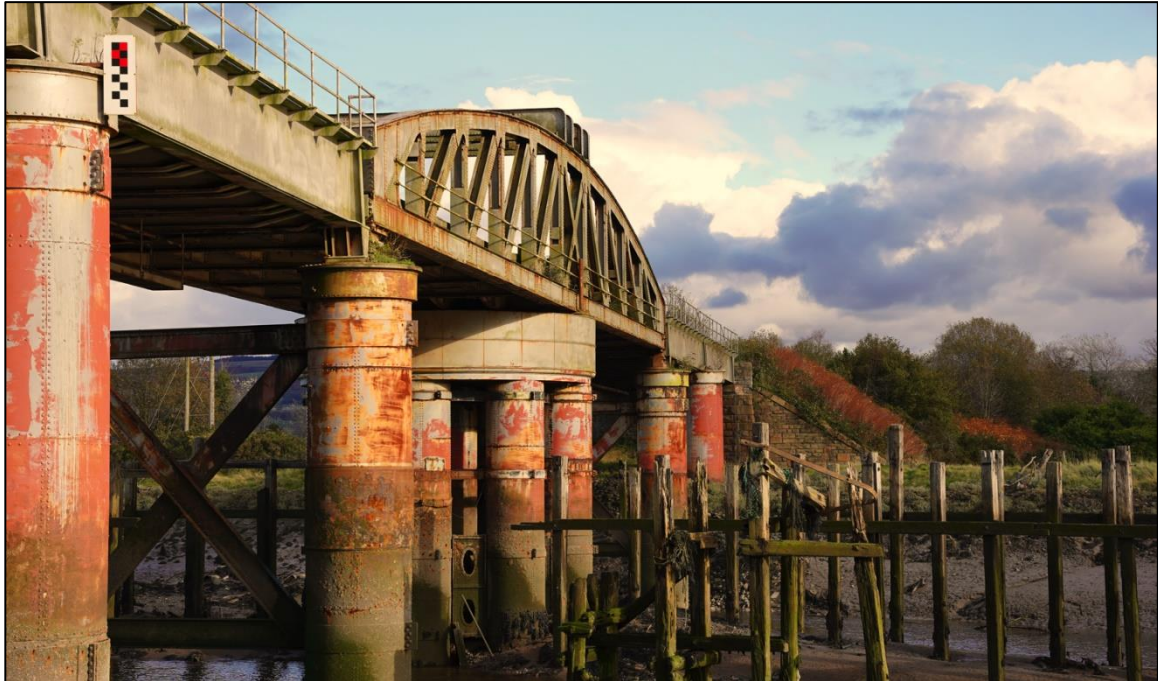
Figure 5: Overview of Neath Swing Bridge from Western Shore (Facing East).
