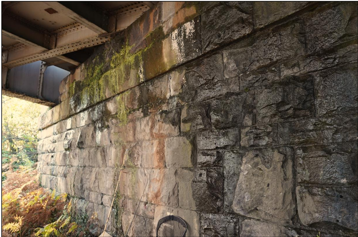
Figure 12: Lower masonry below steel decking.
