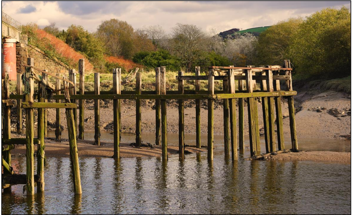
Figure 7: Remaining timber sections from past operational periods.
