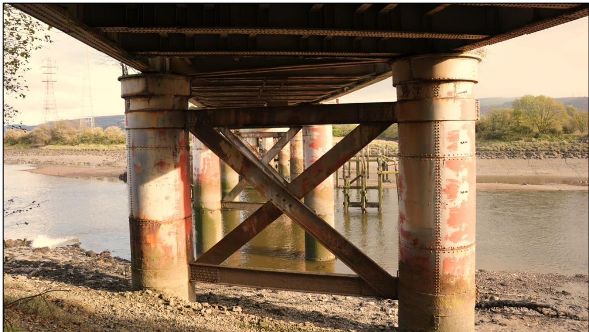
Figure 6: Below space between first and second set of metallic piers.
