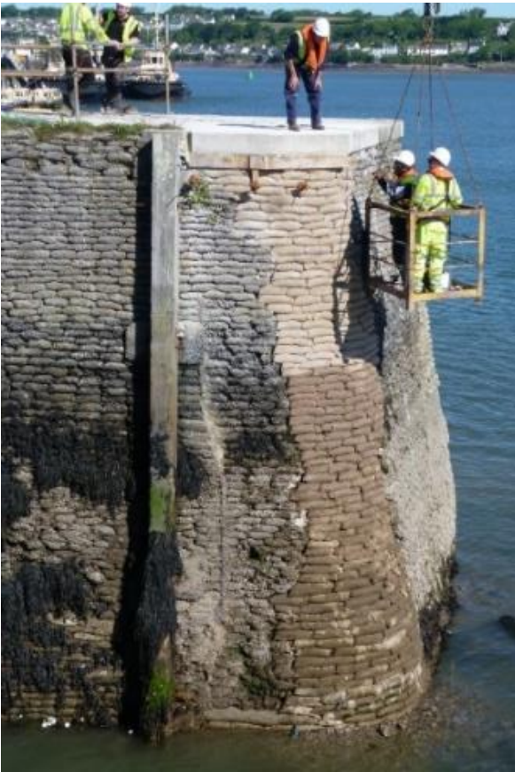
Figure 3-10 Repointing and Wall Repairs by Rope Access
