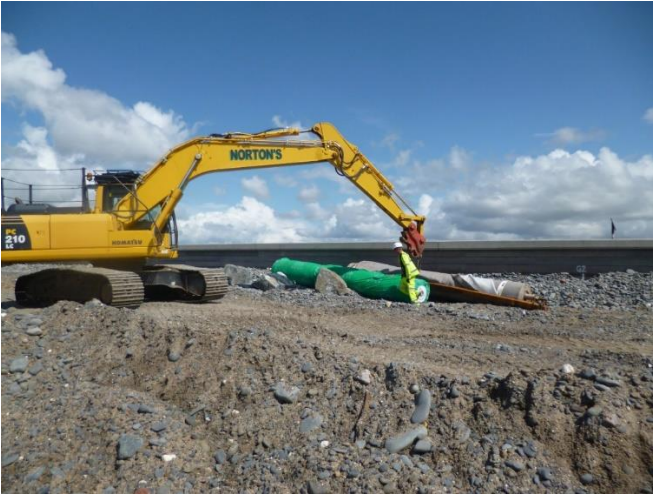
Figure 3-3 Tracked Excavator with Grab for Rock Placement
