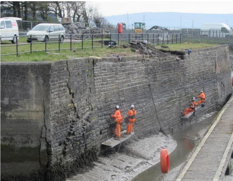
Figure 3-10 Repointing and Wall Repairs by Rope Access
