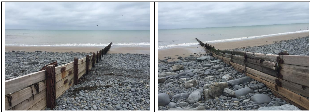
Figure 2-3 - Existing timber groynes on South Beach
