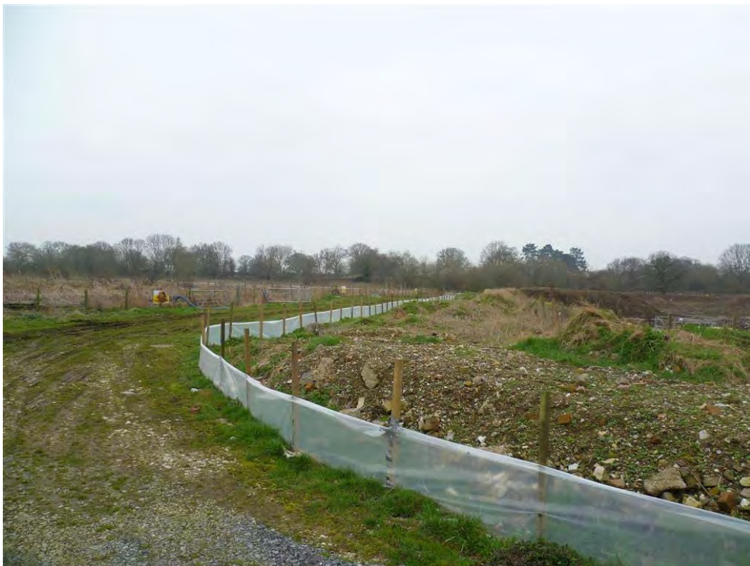
Photograph 4: Eastern boundary of site with new fence looking towards proposed location of thickeners / poly kiosk, odour control and HV and LV distribution kiosk
