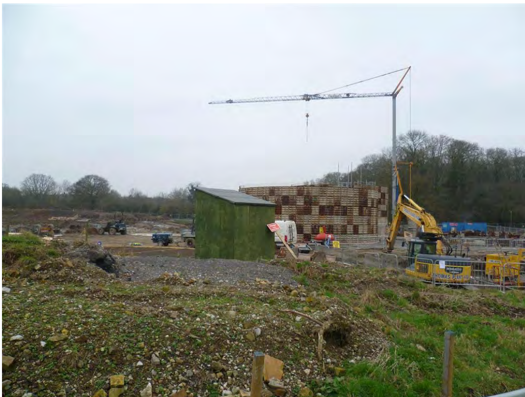
Photograph 6: View from East boundary of site towards digesters and proposed location of gas holder at western boundary
