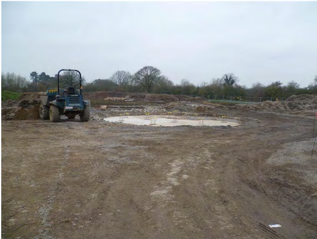
Photograph 1: Proposed location of thickened sludge buffer tank, digester feed pumps and mixer
