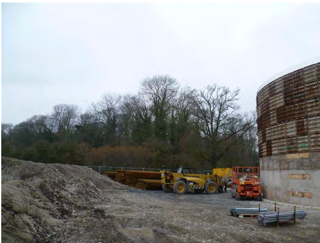
Photograph 2: Location of digester looking towards west boundary of site
