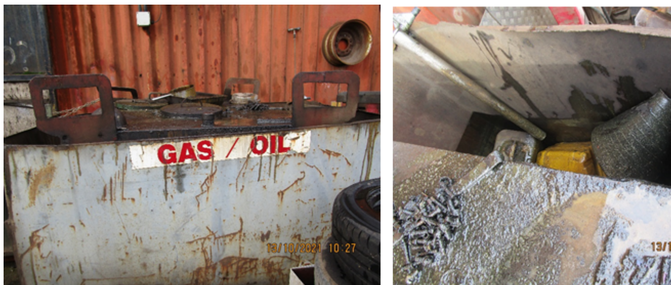
Figure 2. Double bunded waste oil tank containing some items inside the bund.
