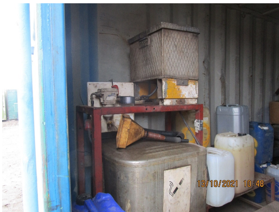
Figure 2. Double bunded waste oil tank containing some items inside the bund.
