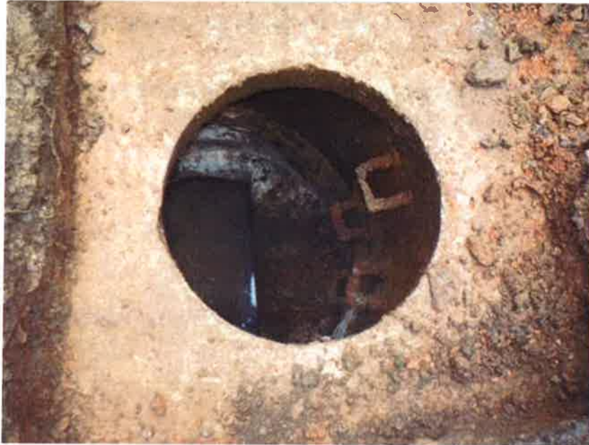
Photo 3: E9 chamber following improvement work
