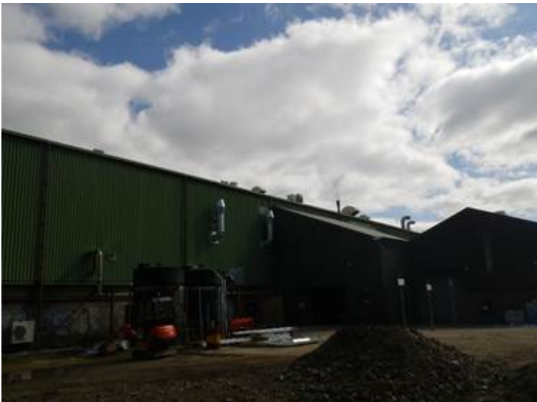
Photo 12: New extraction vents
