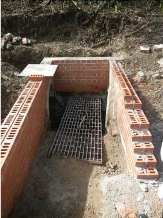
Photo 11: S30 in process of being re-built
