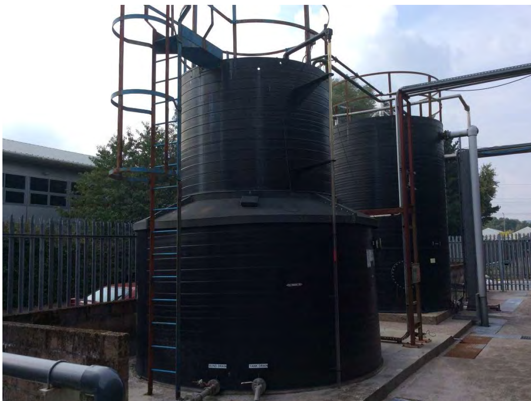
Figure 4.1.1: Photograph of A18 Phosphoric Primary Tank with Collar Bund
