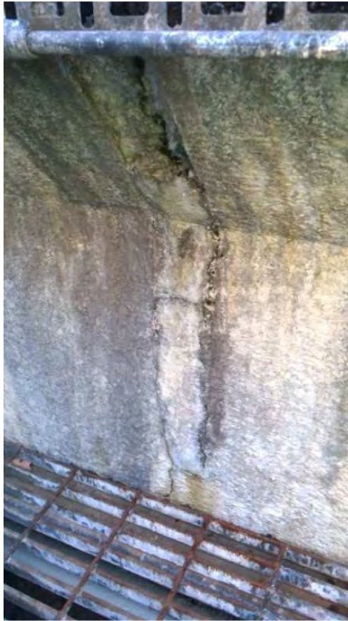
Photo 4.4.6 : Caustic Tank – Contraction joint (2)
