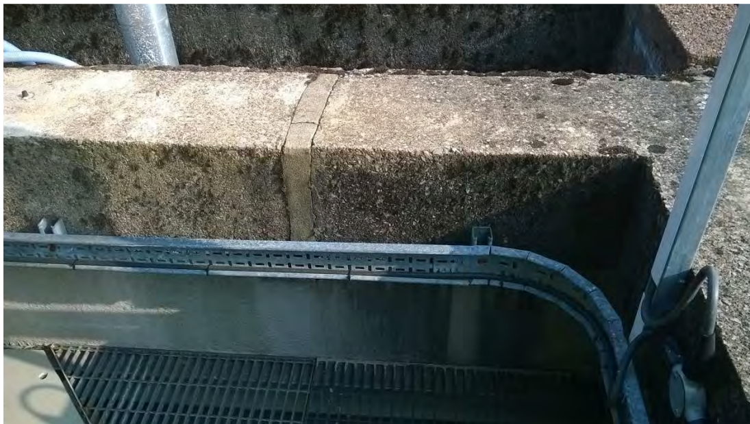
Photo 4.4.7 : Caustic Tank – Contraction joint (3)
