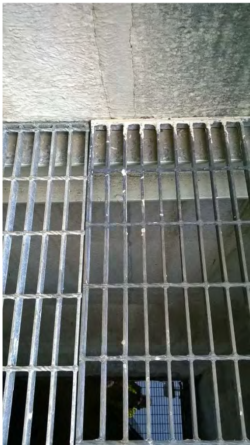
Photo 4.4.5 : Caustic Tank – Contraction joint (1)
