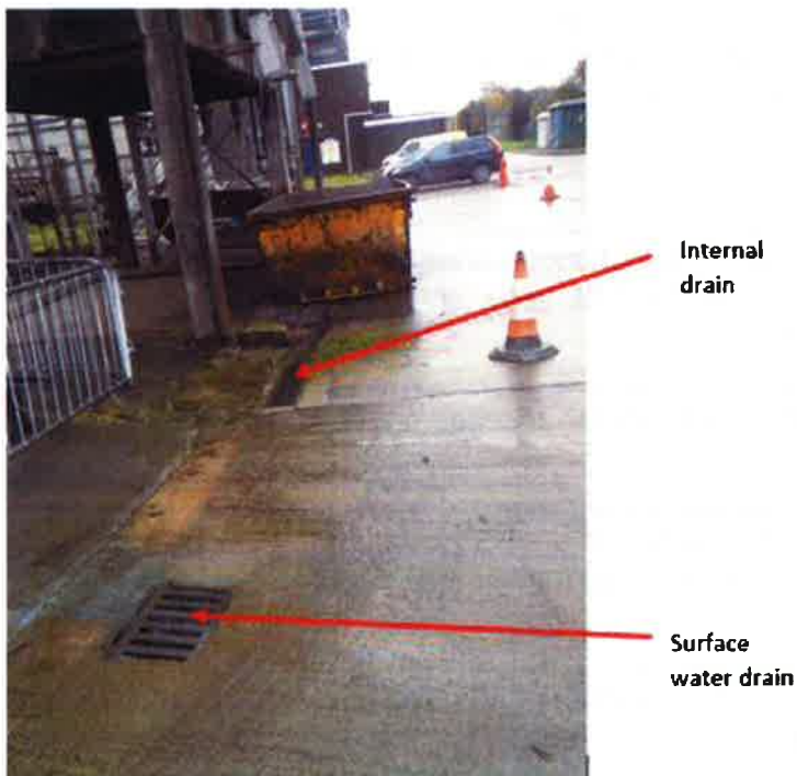
Photo 5: Surface water drain location
