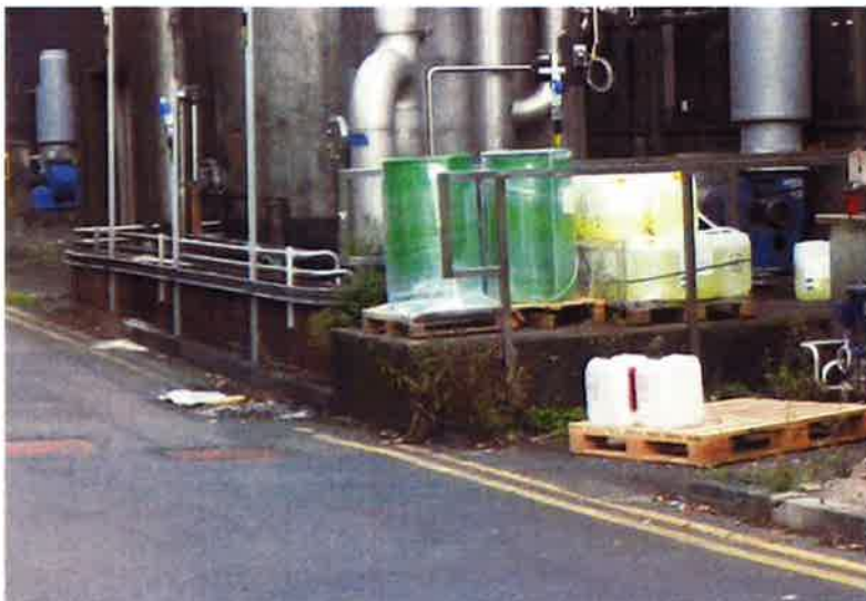
Photo 1: Temporary storage of chemicals
