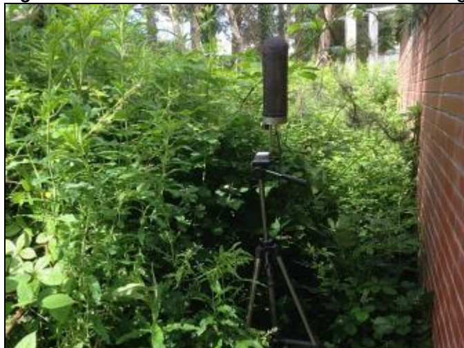
Figure 5: Location 2 at rear of brick sub-station building
