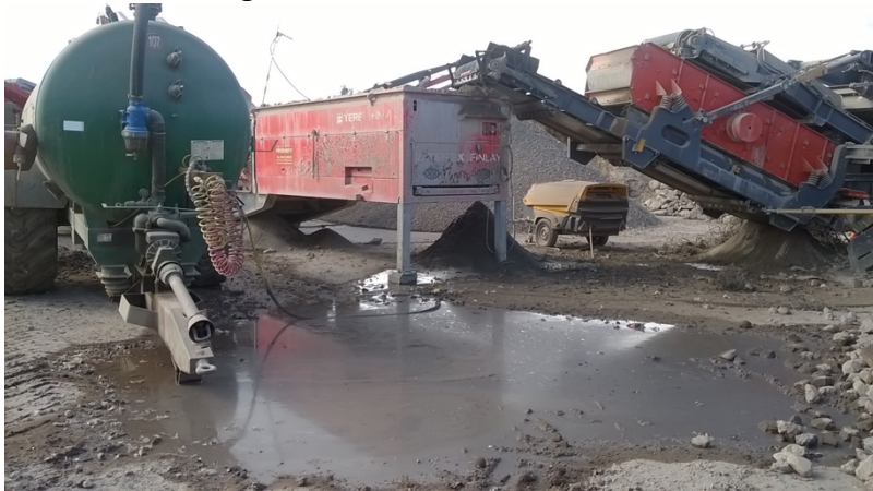
The crusher closed down, evidence of water tanker on site and de-misting equipment.
