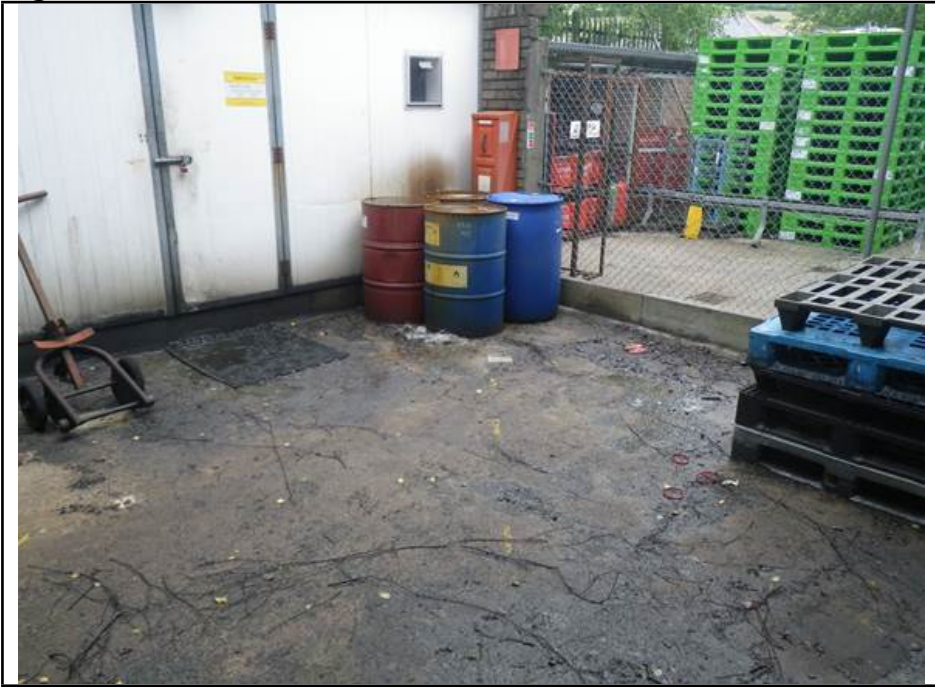
Figure 1: Unsuitable bunded area
