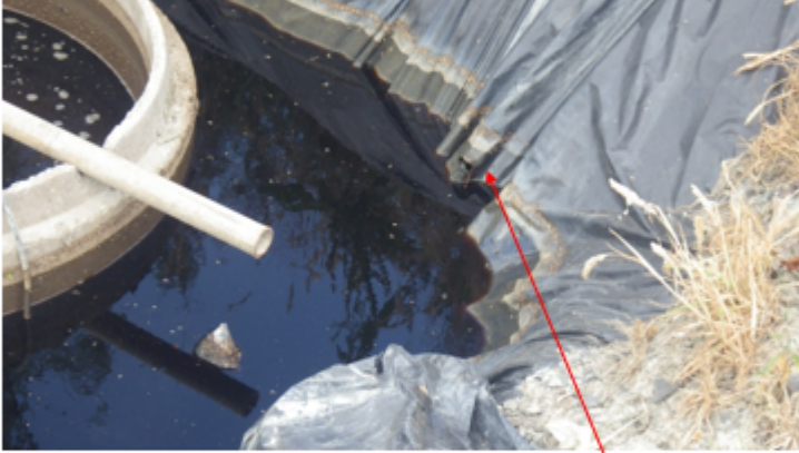
Hole in lining of sump
