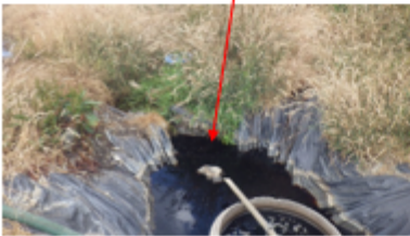
Example of where lining has failed on the sump
