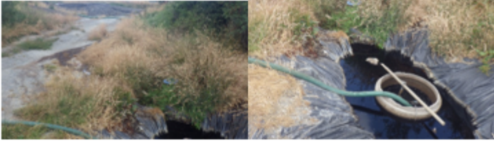
Leachate outbreak from southern bank of Leachate treatment Lagoon | Sump full of leachate
