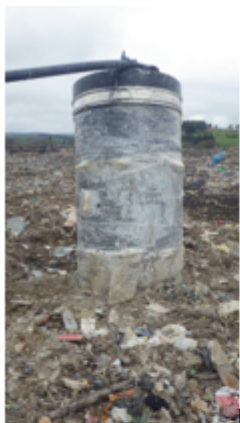
Photograph 2: Attempts made to reduce methane emission from Leachate chambers.
