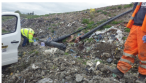
Photograph 3. Repair work on one of the gas collection lines
