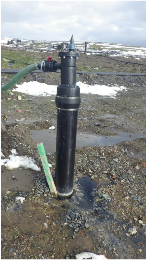
Leachate ponding around base of gas well
