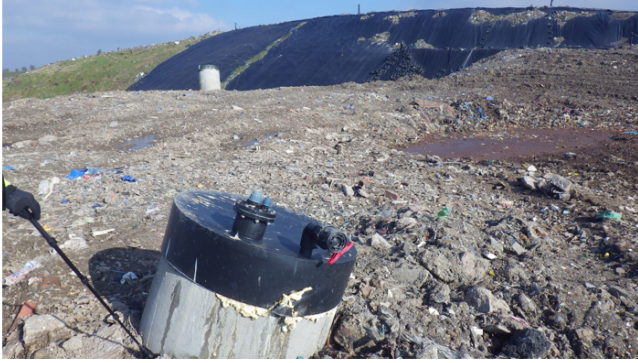
Example of a concrete leachate tower not connected to the gas extraction system.
