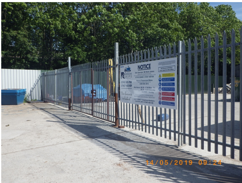
Site gate with ID board
