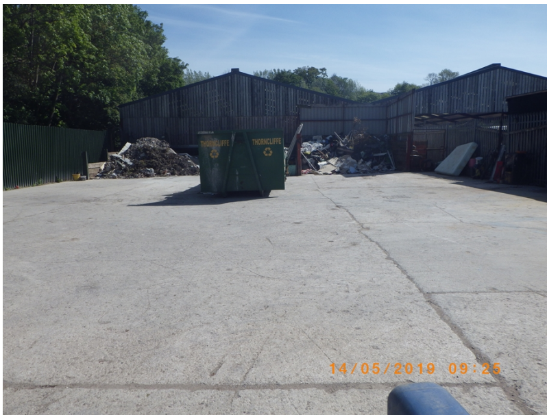
Riverside Skips site (from entrance gate)
