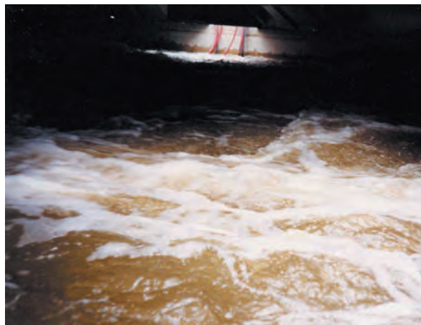
Submersible AirJets in leachate tank
