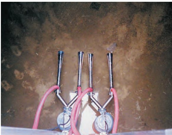
Submersible AirJets in leachate tank
