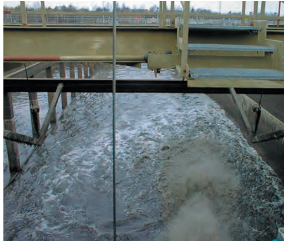
Storm water tank cleaning
