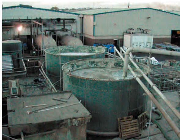
Dry-installed AirJet in tannery effluent aeration tank
