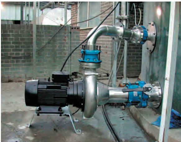
Dry-installed AirJet in tannery effluent aeration tank
