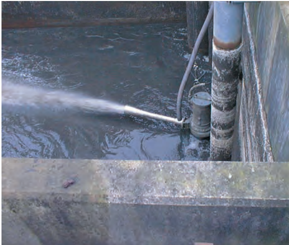
Storm water tank cleaning
