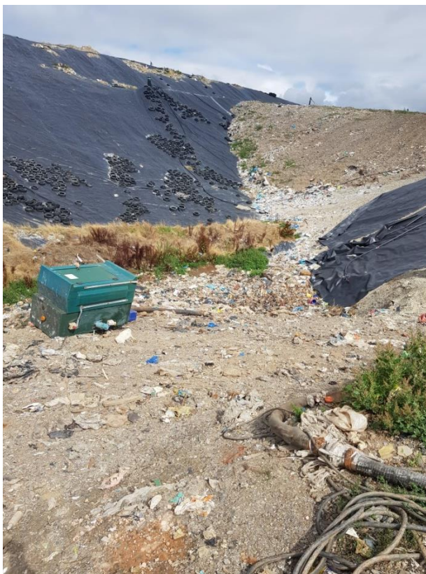
Plate 1; the long and steep southerly facing waste slopes in Phase 9 with the pumped sump at the toe.
