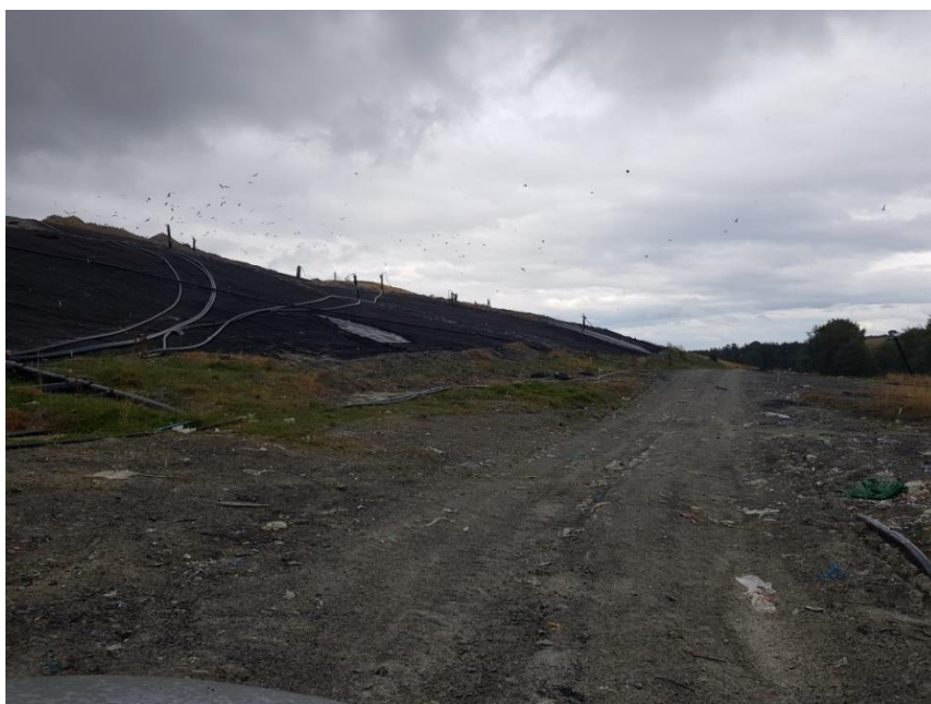
Plate 3; the capped slope to the Eastern boundary of the site covered with the protection geotextile.
