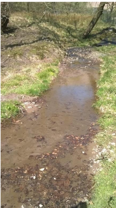
Plate 2: Sediment deposition from upstream works.
