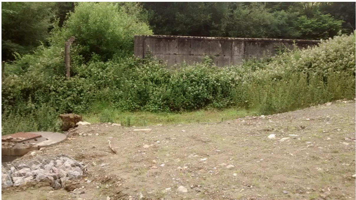
Photograph 7 – Leachate lagoon (view from east)
