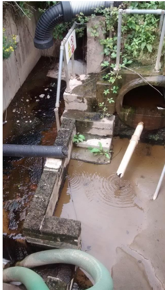
Photograph 2 – Leachate sump inputs
