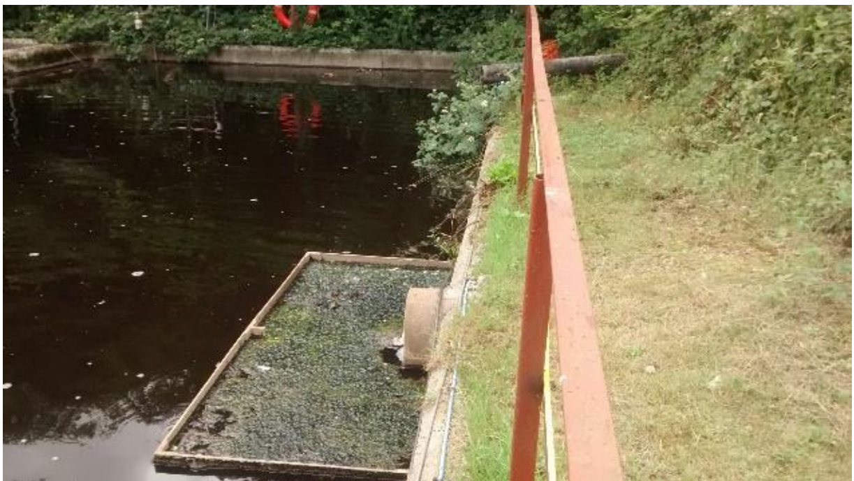
Photograph 5 – Inputs to leachate lagoon
