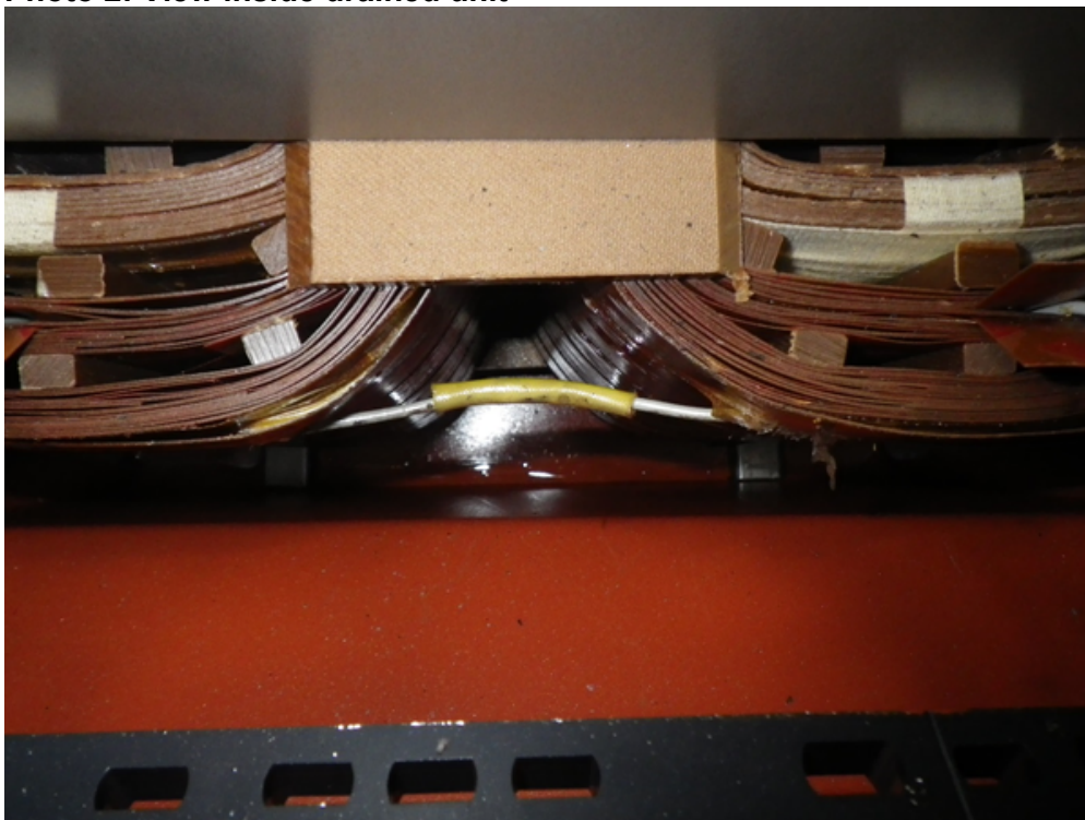
Photo 2: View inside drained unit
