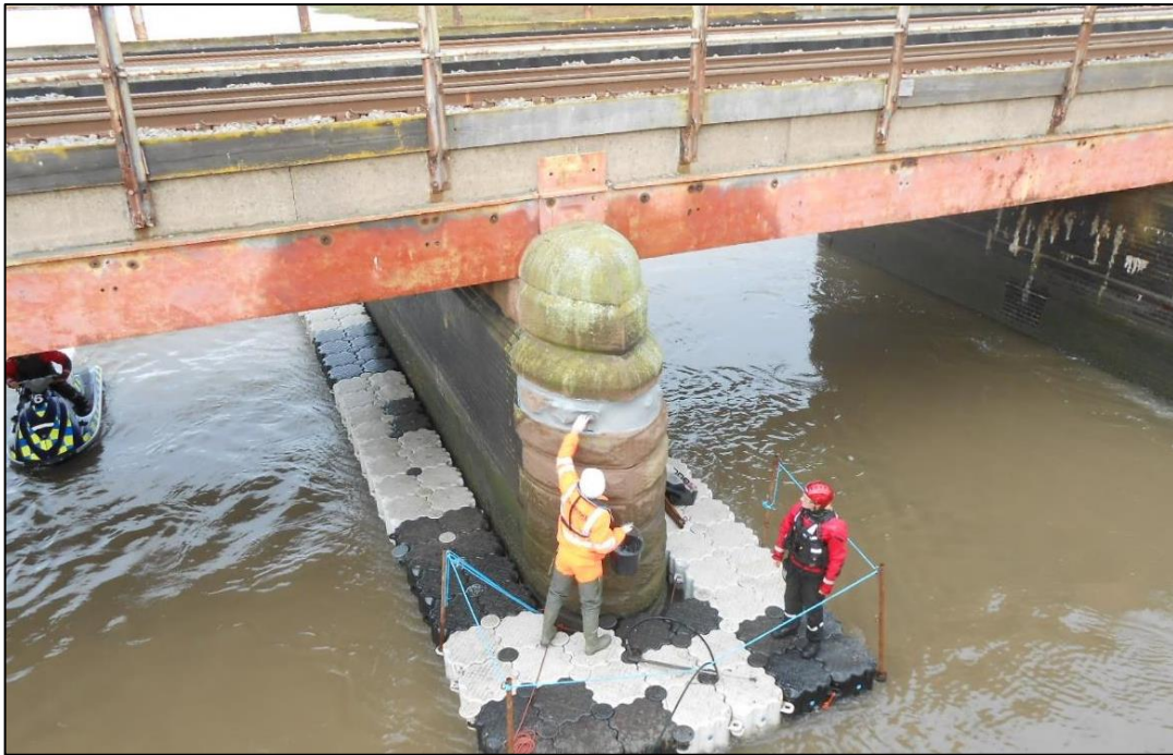
Figure 7: Example of pontoon wrapped around pier.
