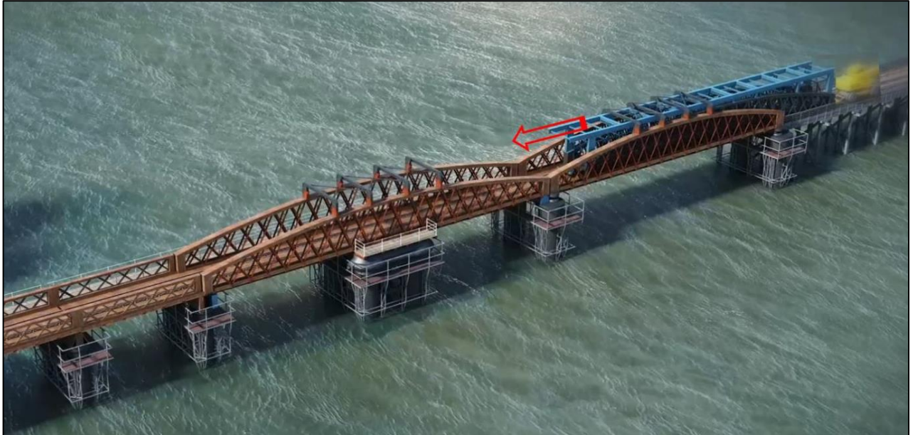
Figure 10: New bridge sections and loading beams driven into space between existing outer frames.
