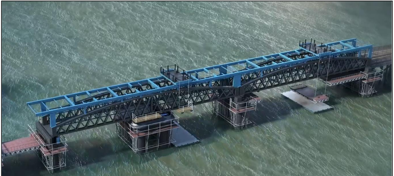
Figure 13: New outer structure supports, and frame widened, and new decking raised and fixed into place.
