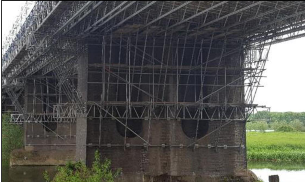
Figure 5: Example of scaffolding above high waterlines.
