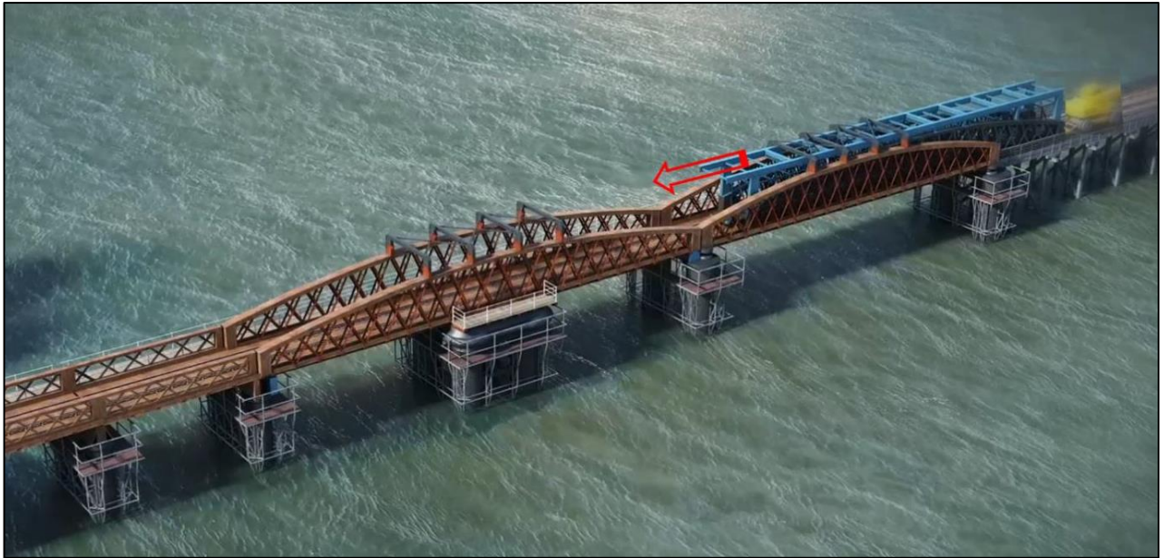
Figure 12: New bridge sections and loading beams driven into space between existing outer frames.
