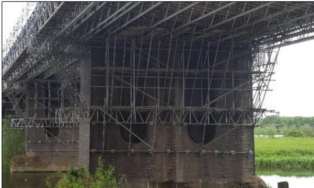
Figure 7: Example of scaffolding above high waterlines.
