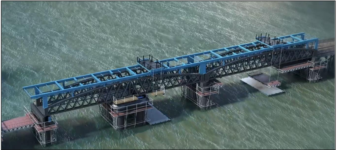
Figure 15: New outer structure supports, and frame widened and new decking raised and fixed into place.
