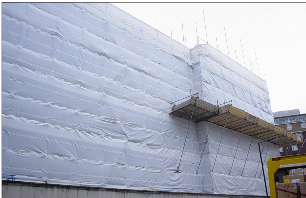
Figure 8: Example of Monarflex sheeting used in an urban setting.
