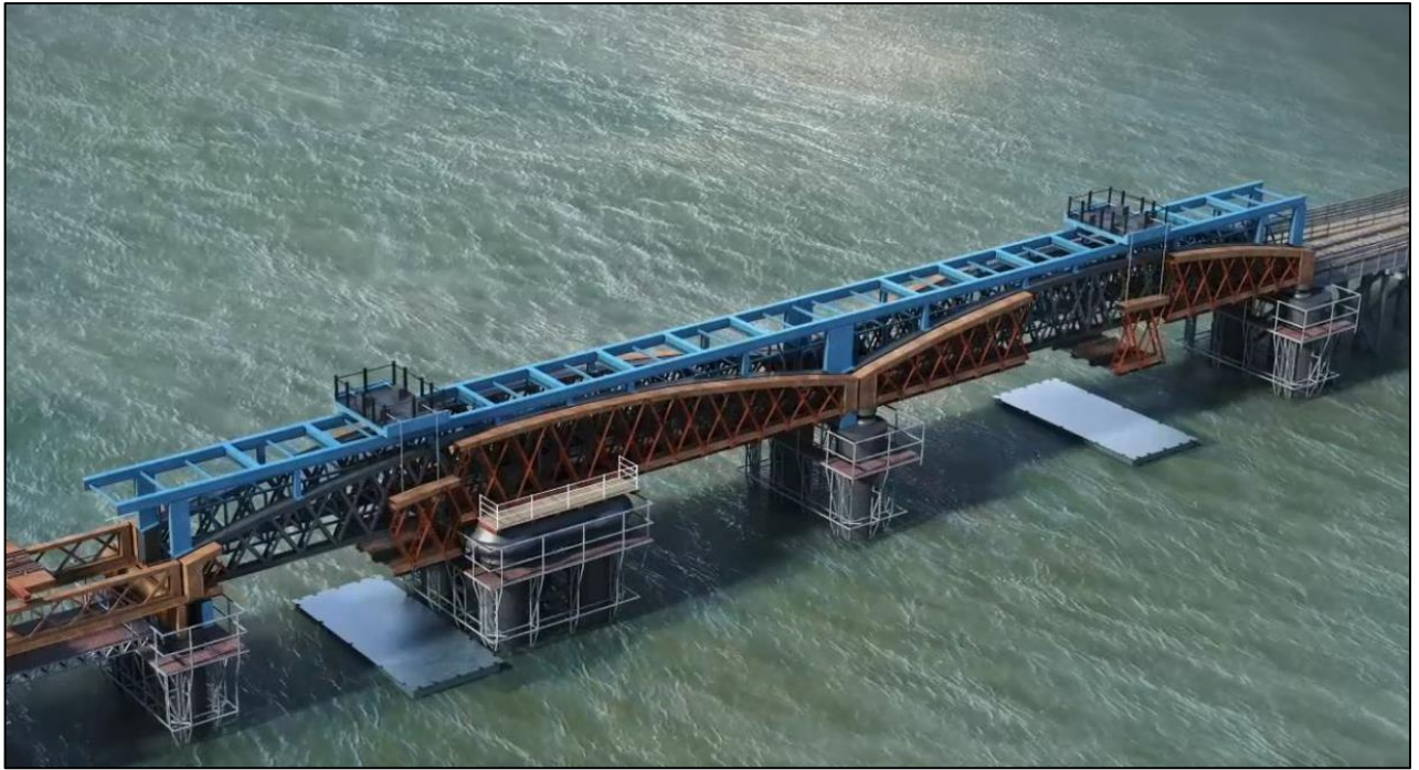
Figure 13: Removal of outer steel work and existing decking.
