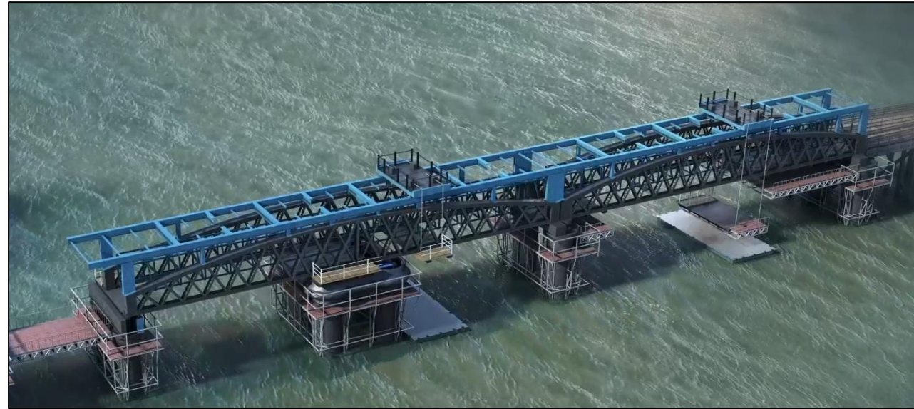
Scaffold around Metallic Section piers and swing section.
