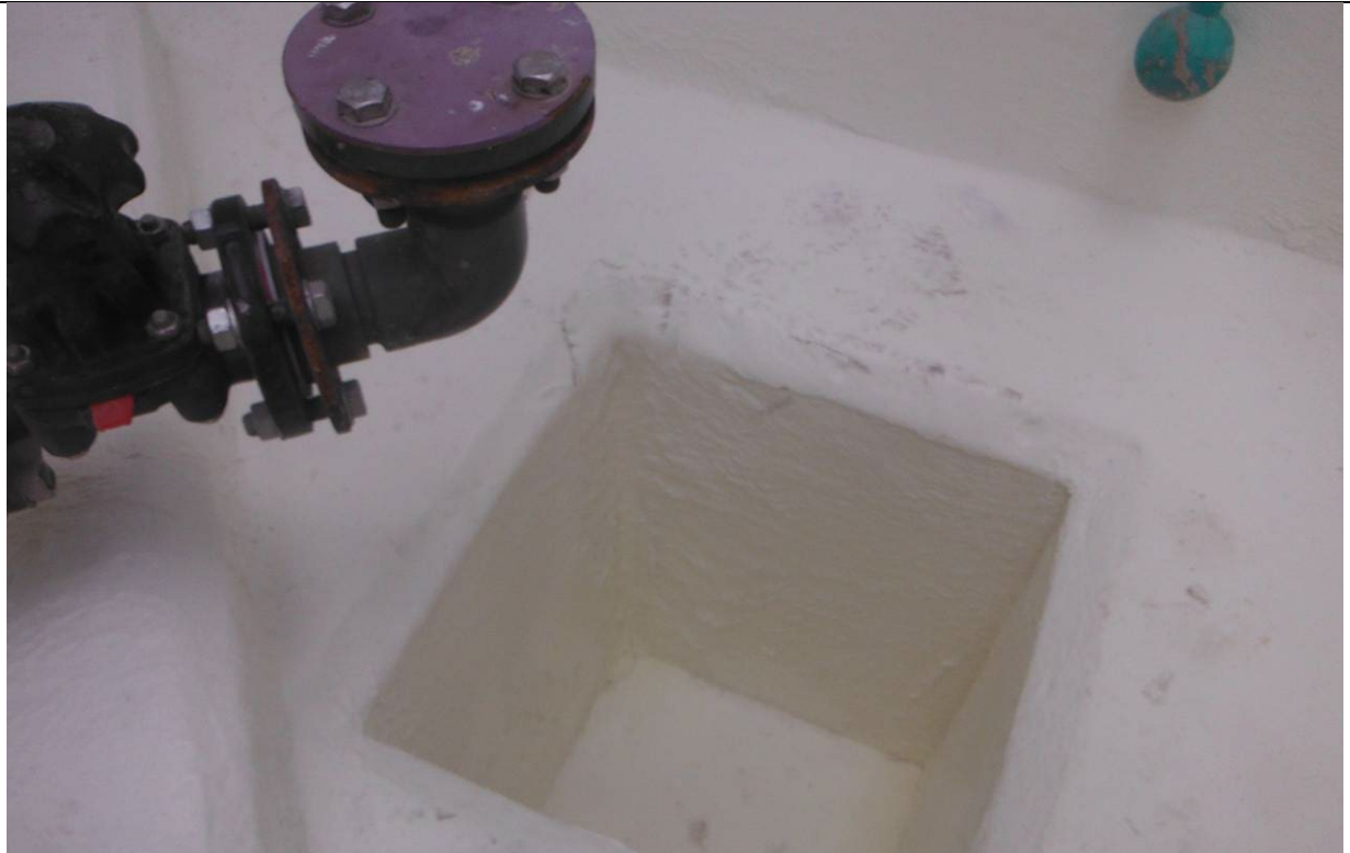
Sump pit with chamfered corners after coating
