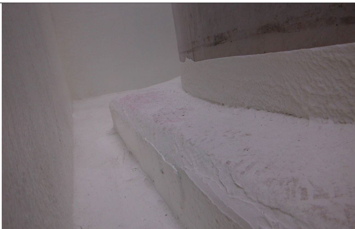
Coating to repaired area of tank plinth
