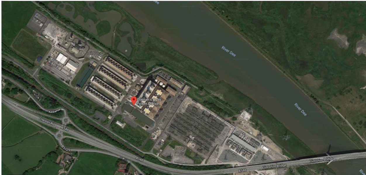
Figure 1: Aerial Imagery of Connah's Quay Power Station (orientation North)
