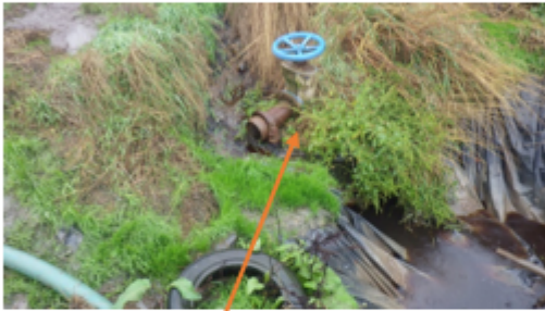
Valve connected to de sludging chamber which will be made redundant together with the de sludging chamber itself.
