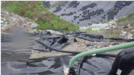
Wind damage caused to some of the emergency works carried out recently
