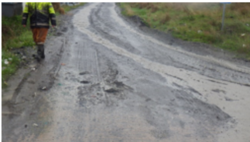
Significantly runoff deriving from site during time of visit, which was entering directly into watercourse
