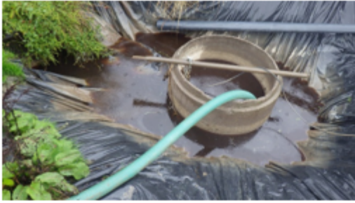
Emergency sump located below the leachate treatment lagoon with escaped leachate still draining into it
