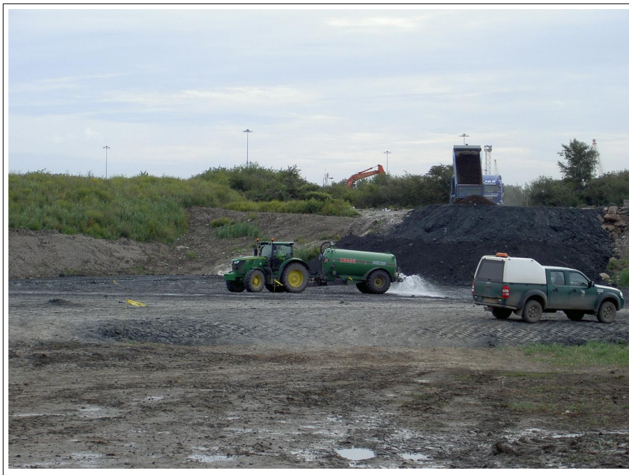
new clay stockpile
