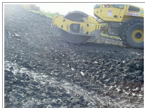
overburden to provide launch for compactor
