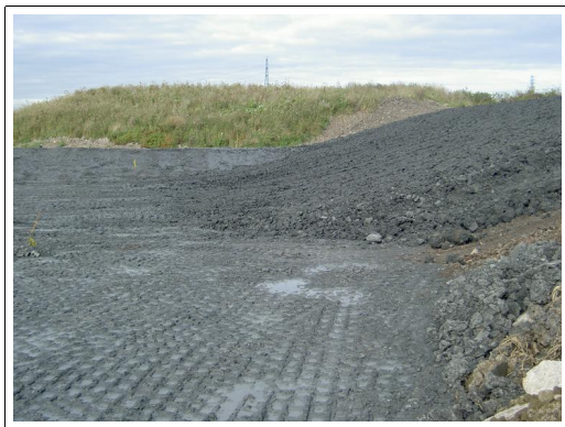
side slope clay, G6 and G7
