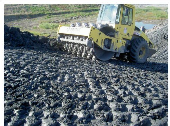
final layers at sideslope (G4)
