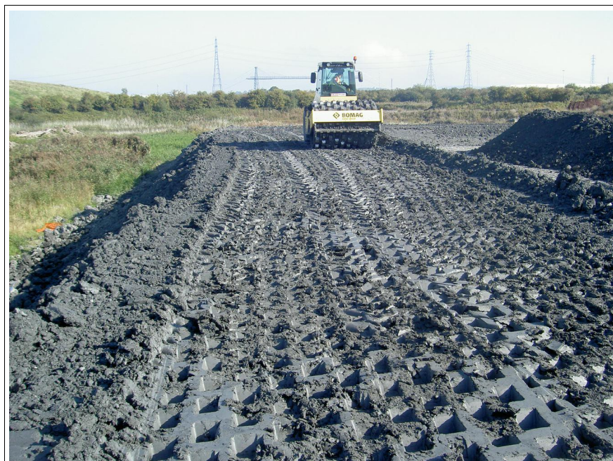
A5, A6, A7 layer 10 scarified, re-wetted and re-rolled
