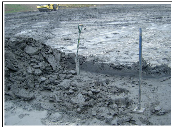
cell excavated to underlying layer
