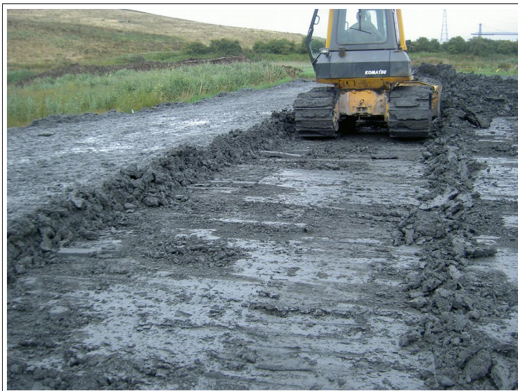
cells D7, B7 and D6 scraped and dried before re-compaction
