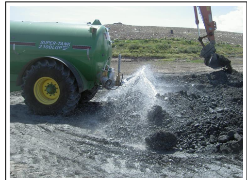
Wetting & conditioning at tipping face
