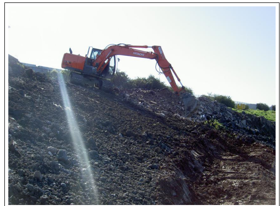
clearing debris from side slopes
