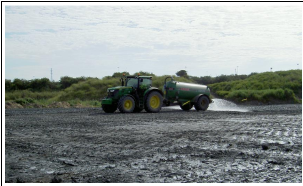
Wetting to maintain condition following compaction
