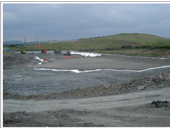
drainage stone & geotextile separating layer
