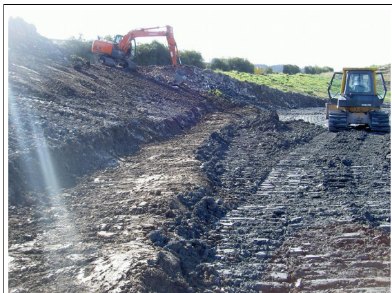
benching at slope bottom, G5, G6
