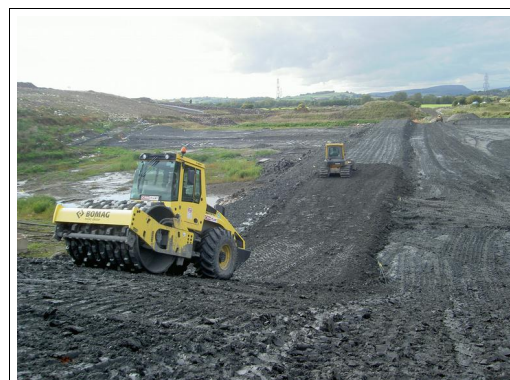
compacting side slopes, G4 (separating bund at row 4 in background)
