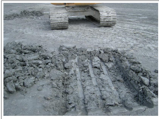
excavating for retests
