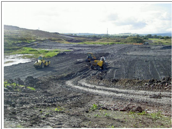
E4, F4, G4 and F5 repairs to bottom of ramp
