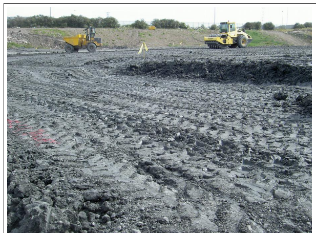
B7 layer 4 excavated
