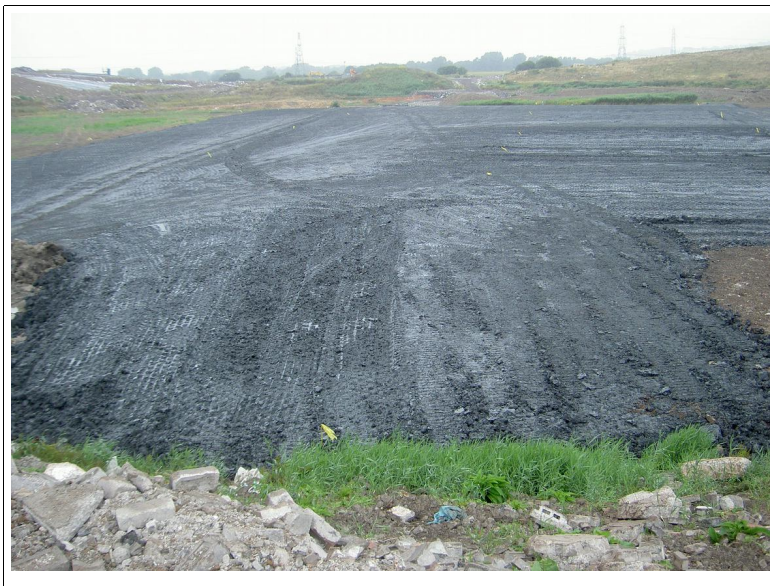
overall progress, Week 4
