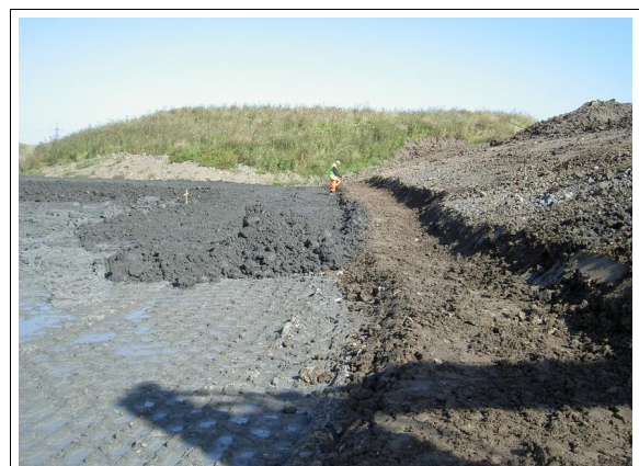
benching at slope bottom, G5, G6, G7
