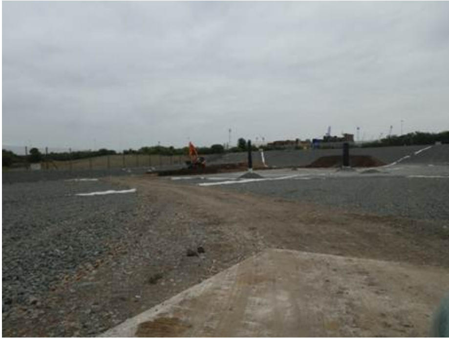
Photo 8: View of asbestos cell from concrete pad where waste arrives
