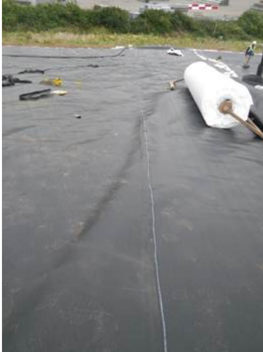
Photo 6: Spreader bars resting on membrane
