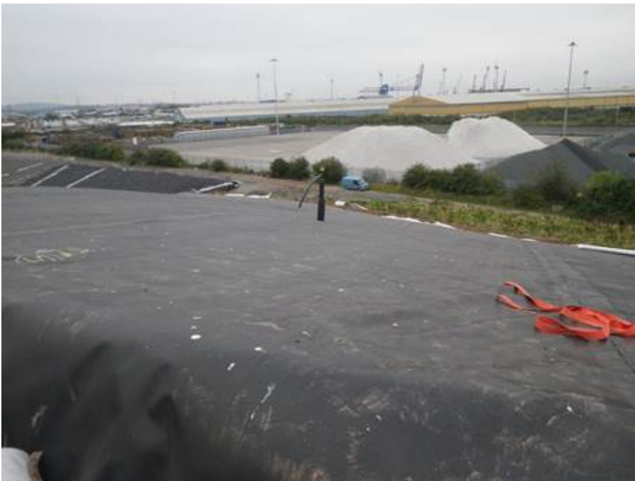
Photo 2: View along capped east flank
