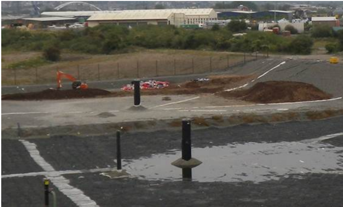
Photo 7: Asbestos waste accepted to site prior to being covered
