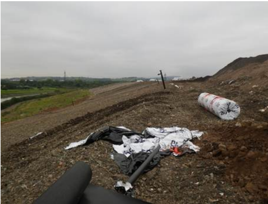
Photo 3: View west along flank to be capped over the laid regulation layer
