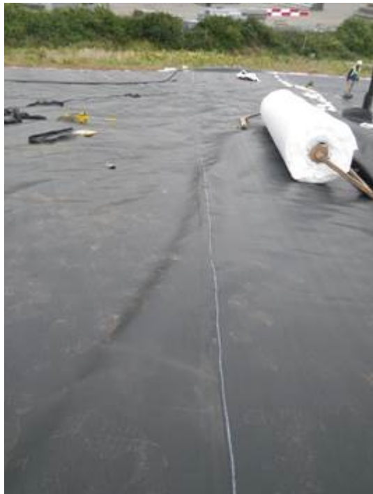
Photo 6: Spreader bars resting on membrane
