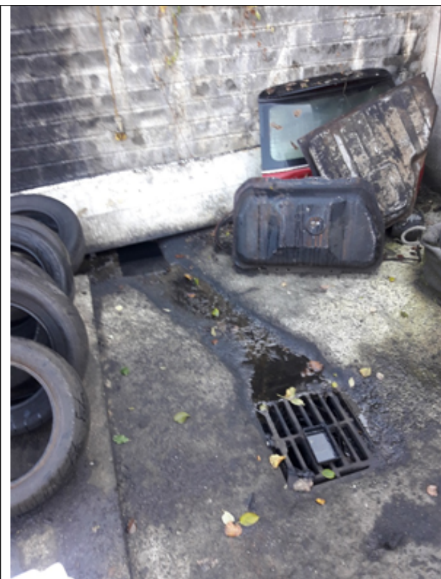
Photo Five - Oil staining on entrance gully
