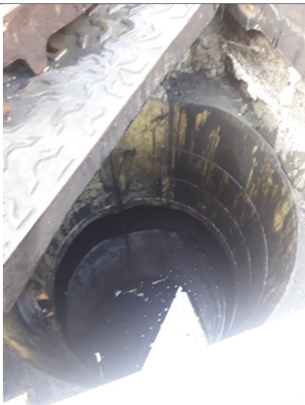
Photo Six - Oil staining of interceptor tank
