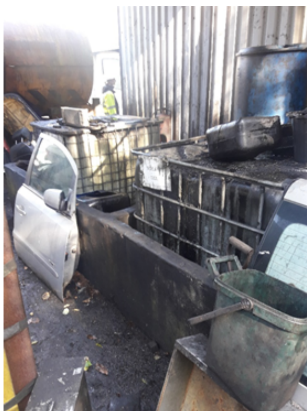
Photo Six - Oil staining of interceptor tank
