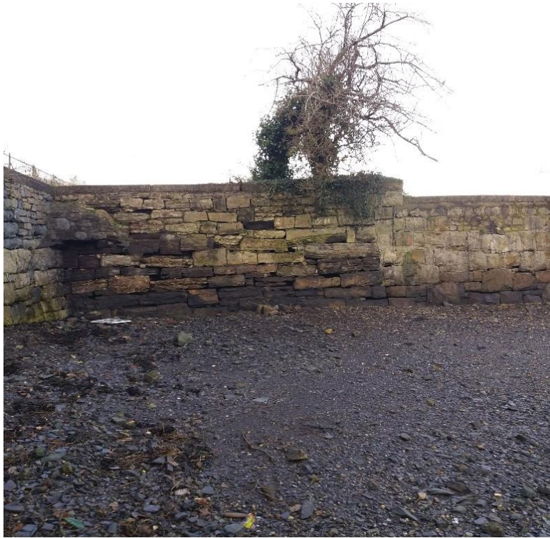
Photograph 5. Existing sea wall to the east of the survey area with slate waste foreshore
