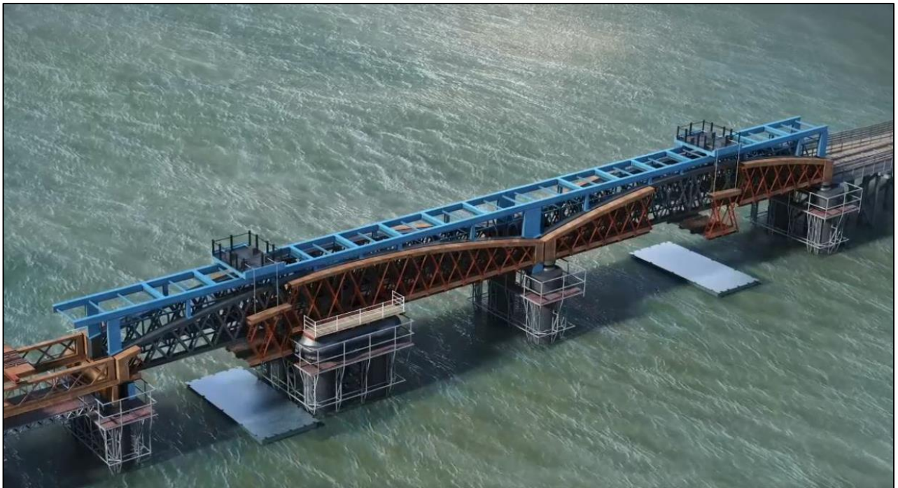
Figure 11: Removal of outer steel work and existing decking.
