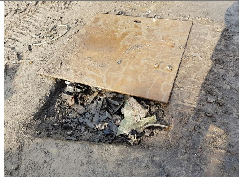
This is in contravention with permit condition 2.3.1 Table 2.3 Operating Techniques, Point 1 which states; All other waste shall be stored on an impermeable surface with sealed drainage system. The clearance and ongoing maintenance of this drain has been highlighted for action and a period of three months has been given for it's completion. Please contact me if this is not achievable.
