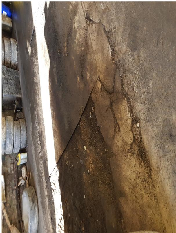
This is in contravention of permit condition 2.3.1 Table 2.3 Operating Techniques, Point 6 which states; All waste shall be treated on an impermeable surface with sealed drainage system. The repair of this concrete pad has been highlighted for action and a period of six months has been given for it's completion. Please contact me if this is not achievable.
