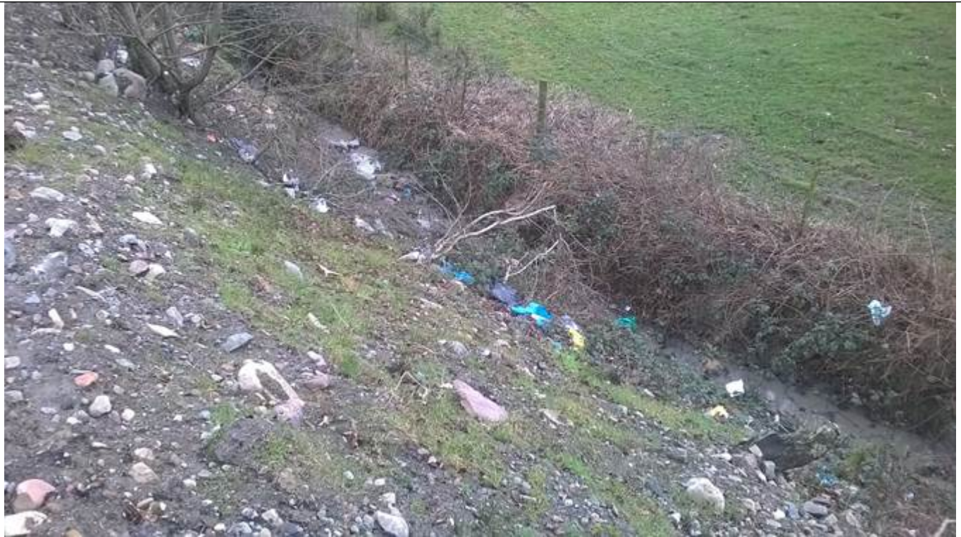
Photo 5 showing resultant high suspended solids in the stream (collected site surface water all passing through a single hydroblock shown in photo 4, and which required urgent cleaning). Note also wind-blown litter
