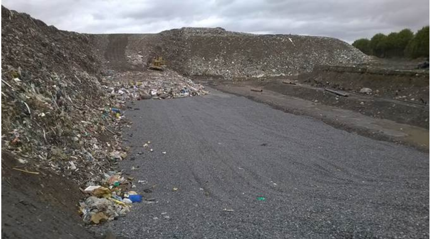
Photo 1 showing tipping access from cell2 to sub cell 5. Note excess wastes from cells 3 and 4 to be moved immediately.
