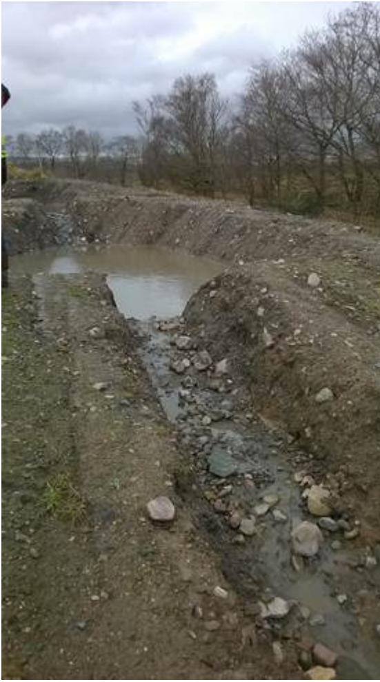
Photo 3 showing unlined channel (design to be improved) accross balancing lagoons.
