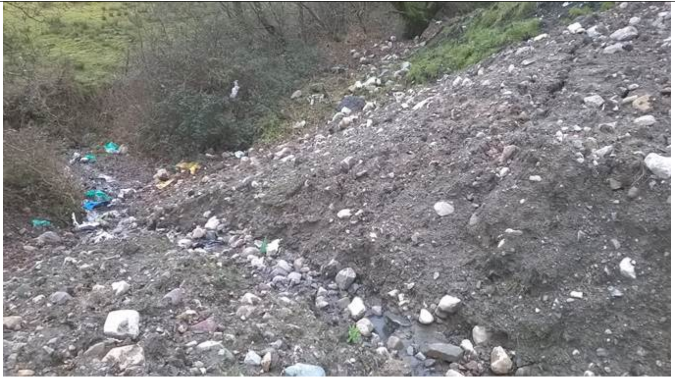
Photo 2 showing tension cracks, silt channel and loose litter above stream
