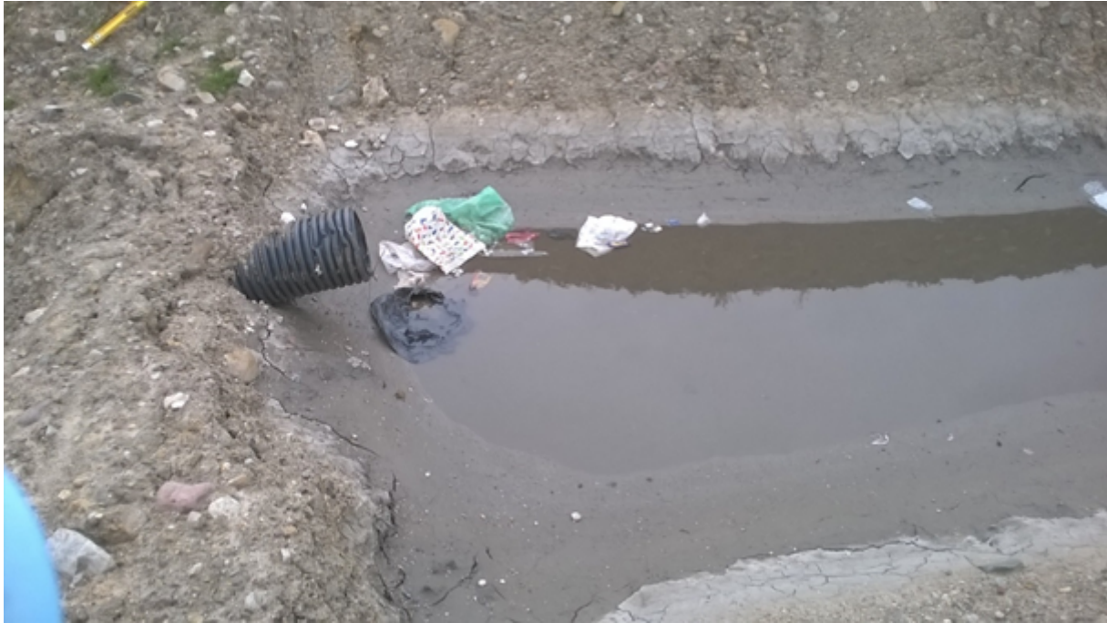
Photo 4 showing temporary sump for valley infill. Note that some sedimentation is taking place, however further improvements can be made fairly easily.
