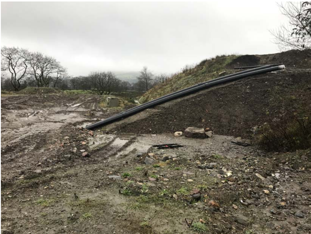
Plate 1. Leachate riser pipes being extended through valley infill
