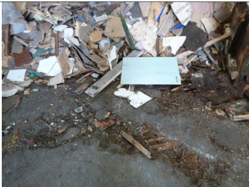
Photo 3. Drainage tank inspection hatch somewhere under waste.
