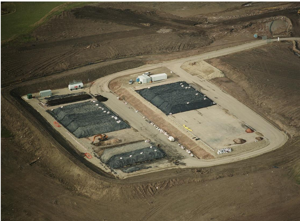
Figure 3-1 Aerial view of the WTF at Biffa's Risley Landfill Site
