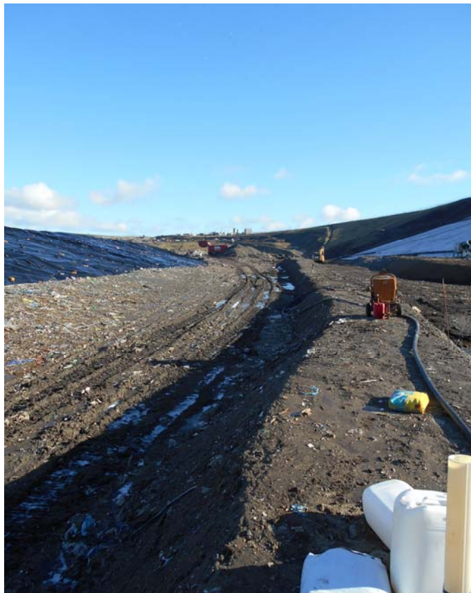
Photograph 8 – Inclinator 1 location looking east.
