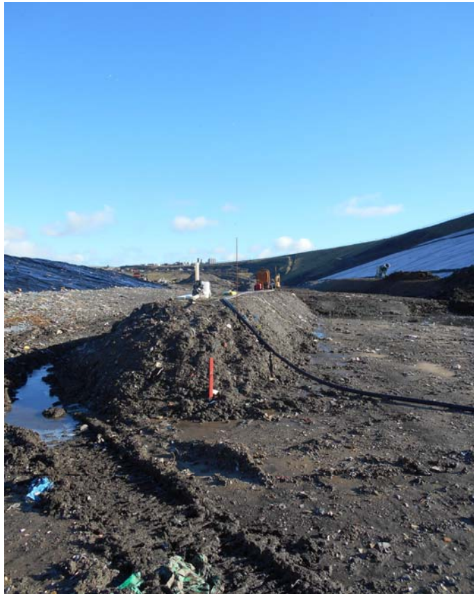
Photograph 7 – Western end of separation bund Lift 3 looking east. SNRHW side
