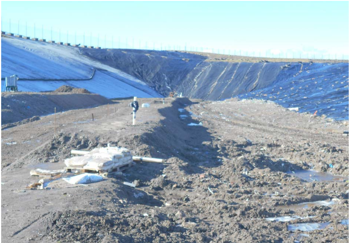
Photograph 1 – Looking west along the completed Lift 3 with Inclinator 3 in the foreground
