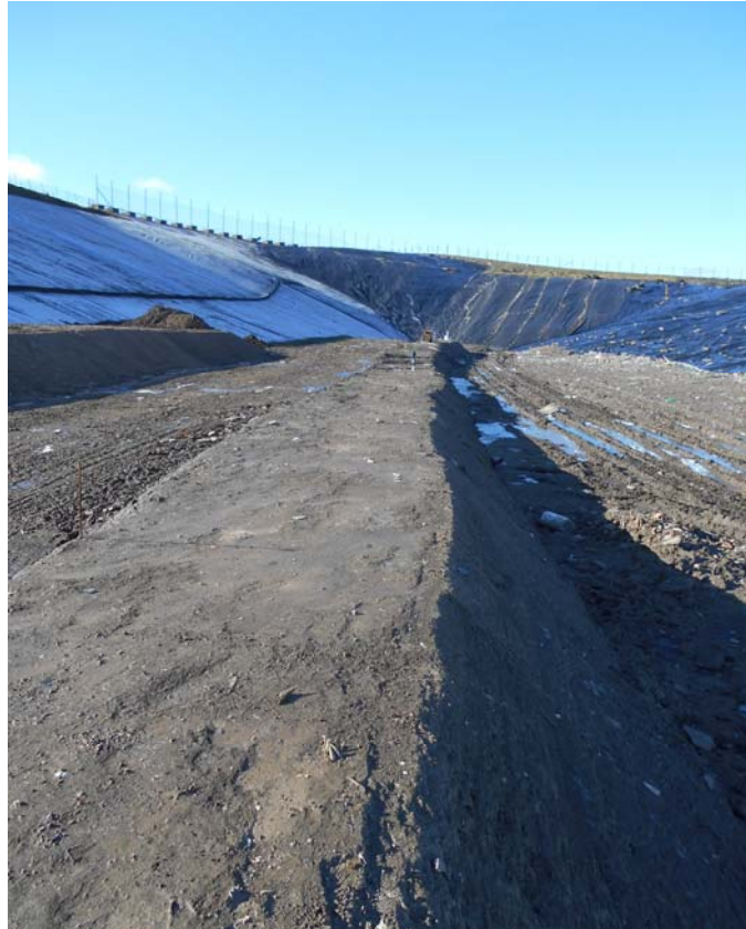
Photograph 3 – Looking west along the completed Lift 3 section of bund
