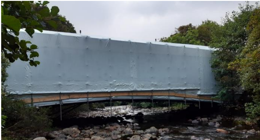
Figure 2 – Example of bridge encapsulation
