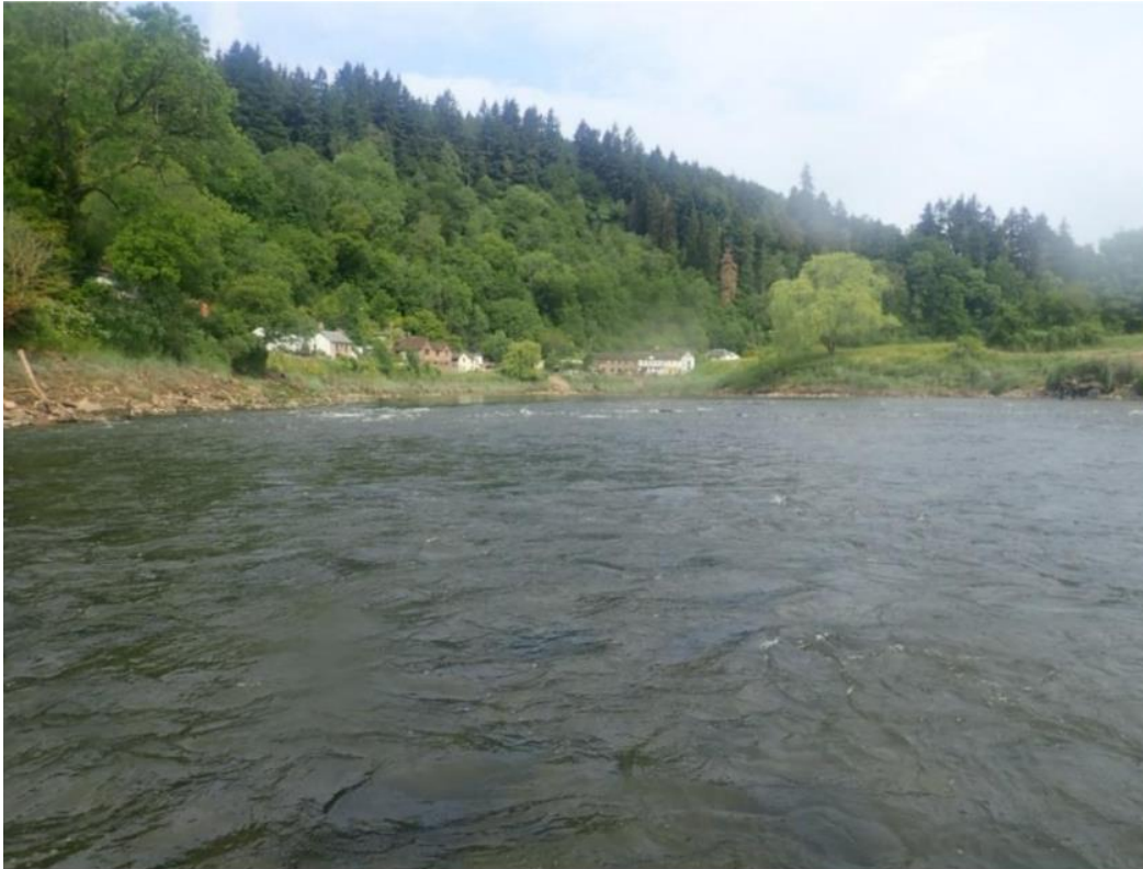
Photograph 3. View upstream of Tintern Wireworks Bridge
