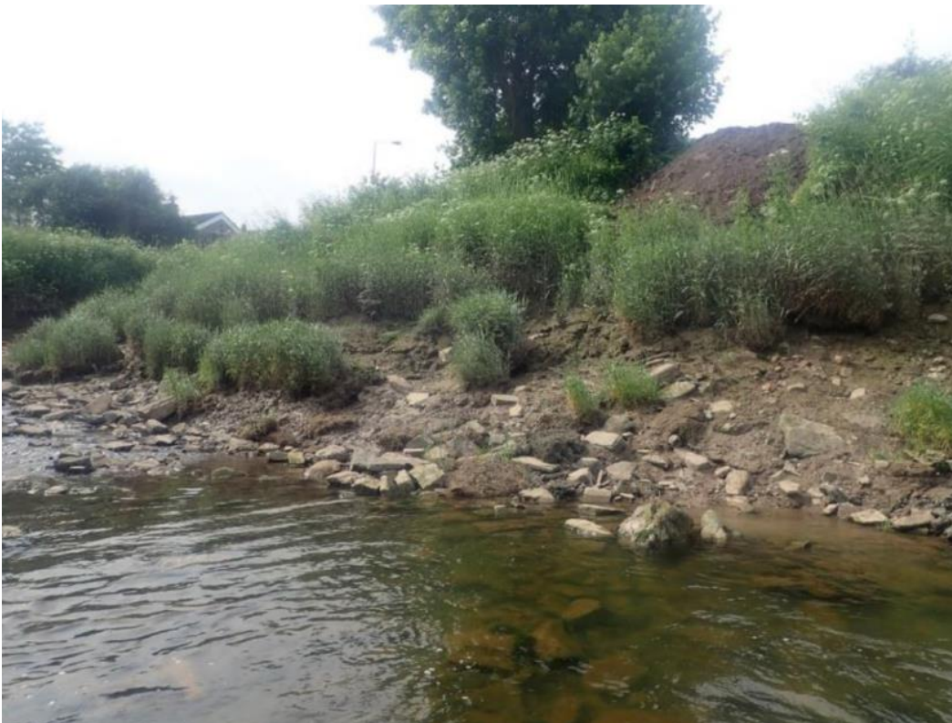
Photograph 6. View of downstream west bank
