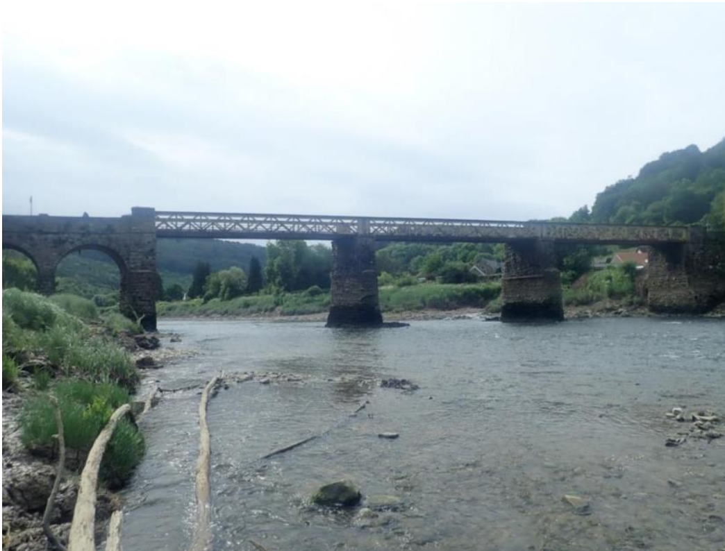
Photograph 1. Upstream elevation of Tintern Wireworks Bridge
