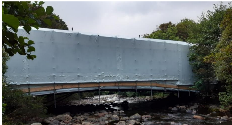
Figure 7 – Examples of encapsulation of a bridge over a watercourse
