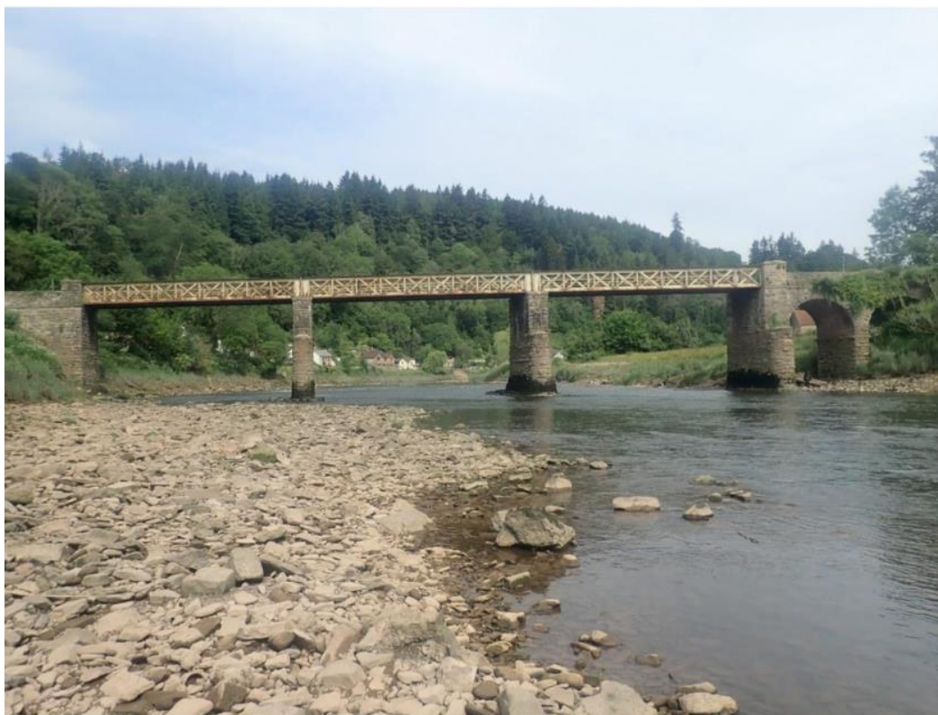
Photograph 2. Downstream elevation of Tintern Wireworks Bridge
