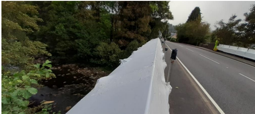
Figure 8 – Examples of encapsulation of a bridge over a watercourse.
