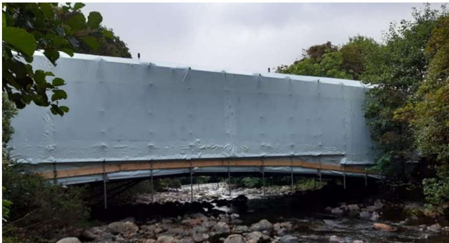
Figure 2 – Example of bridge encapsulation
