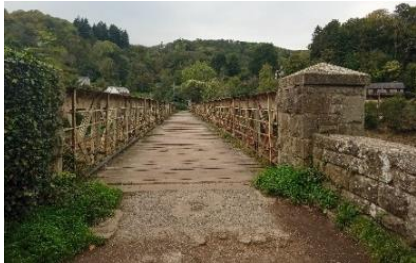
Photograph 2 – The deck of Tintern Wireworks Bridge
