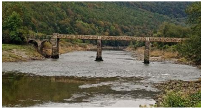
Photograph 1 – Tintern Wireworks Bridge with the River Wye running beneath
