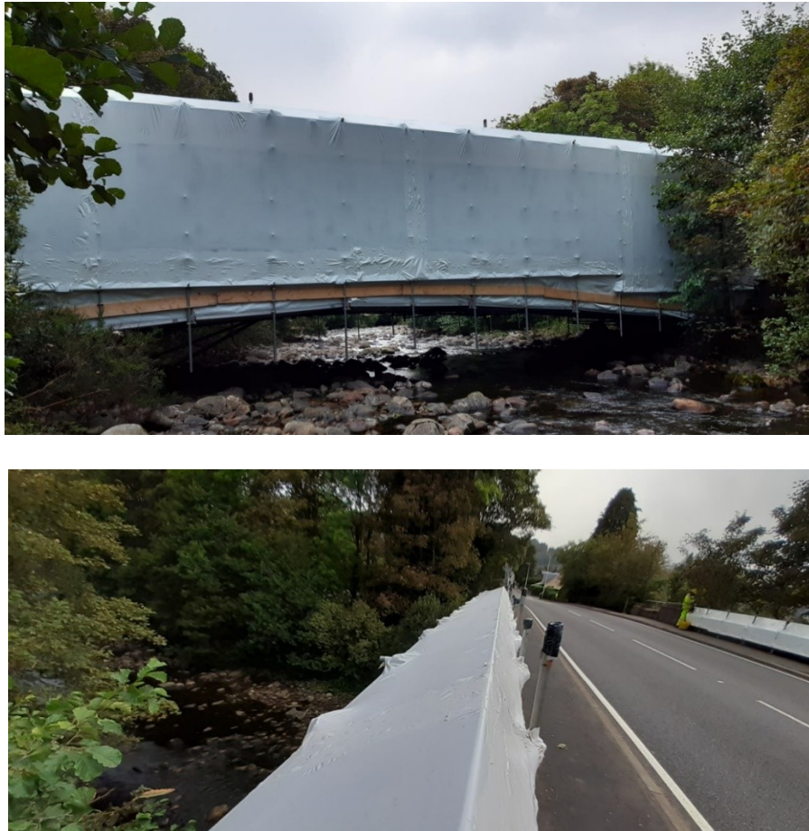
Figure 7 and 8 – Examples of encapsulation of a bridge over a watercourse.
