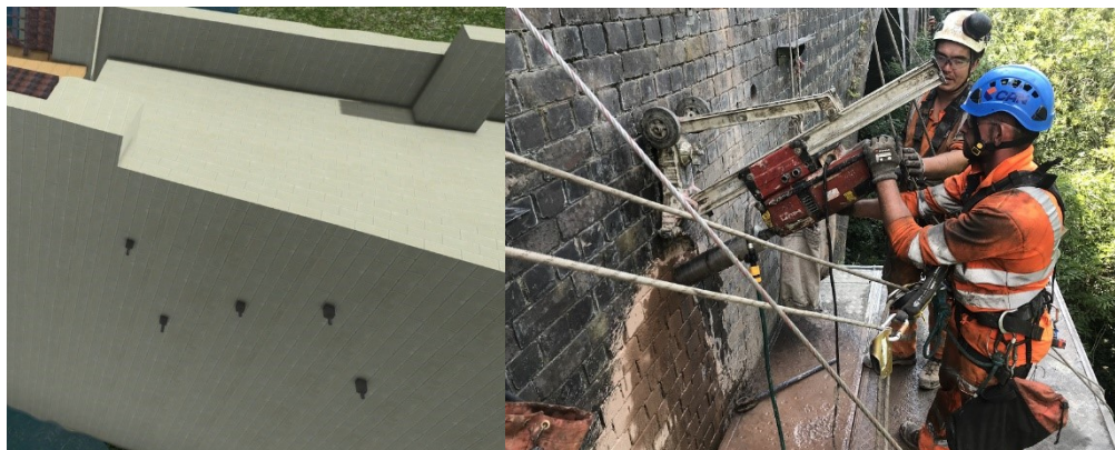
Figure 5 and 6 – Proposed visualisation of the pattress plate system (left- pattress plates are not shown) and examples of proposed method of works (right)
