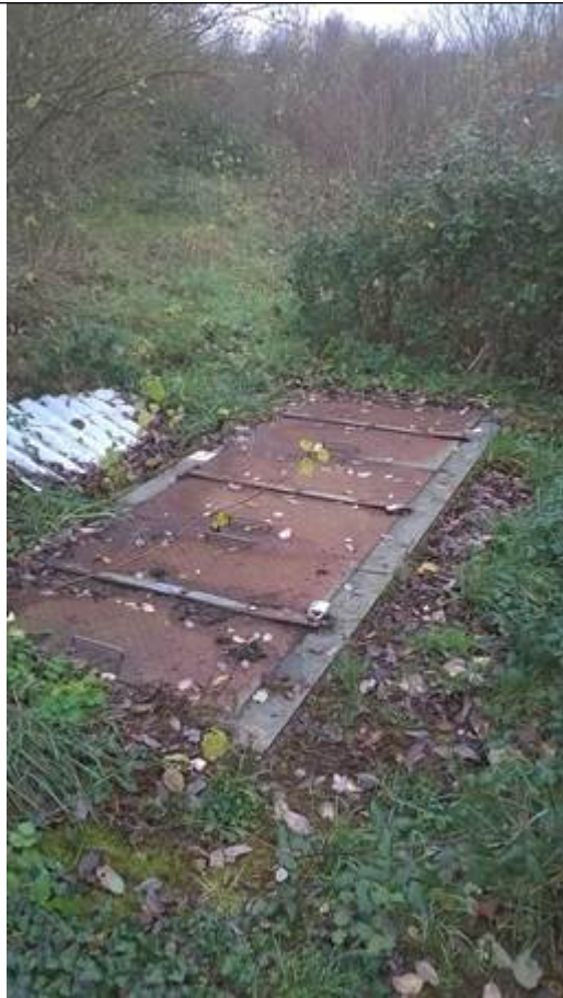
Photo 4 showing gas extraction manifold cover
