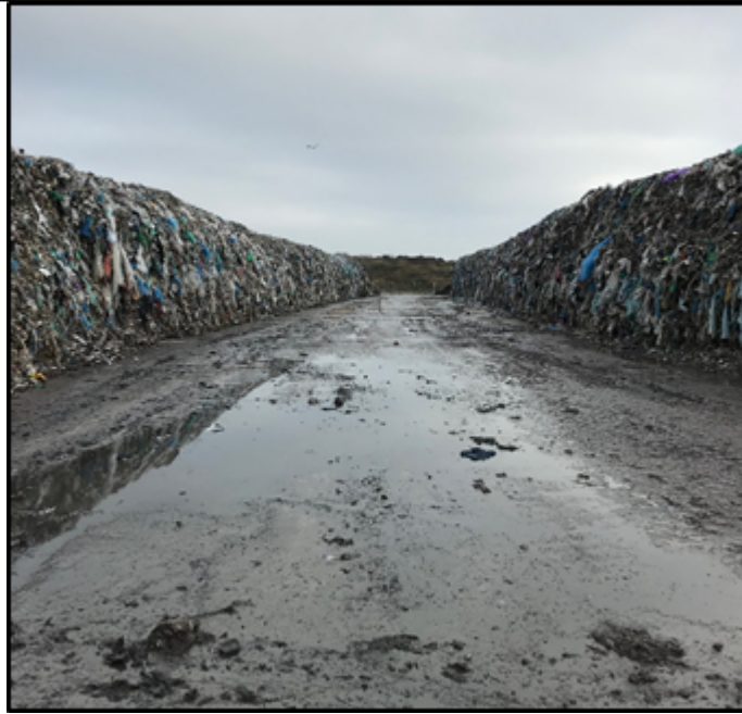
Picture 3 – showing the curbing and net fencing erected around the Transfer Station next to Stockpile 1
