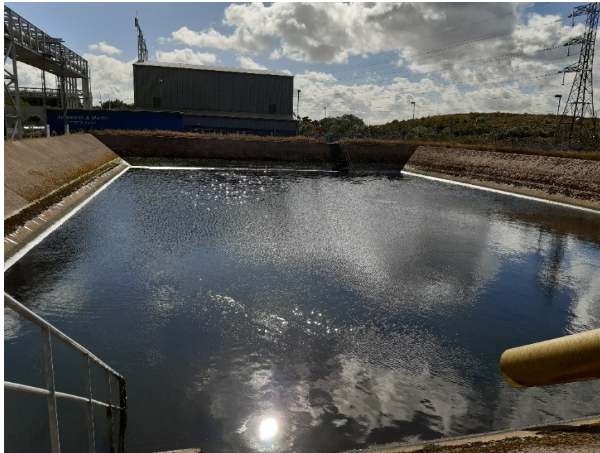
Photo 9. Surface water run-off holding pond
