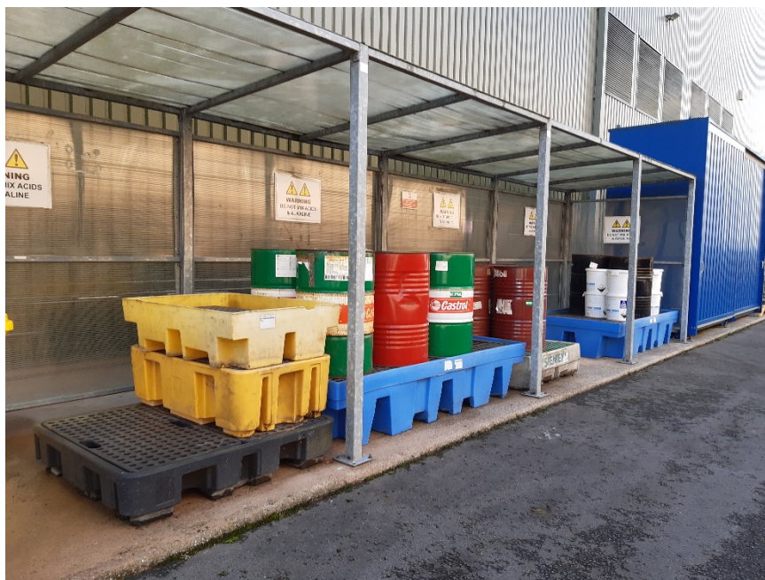
Photo 5. Drum storage of oils, acids and alkalines
