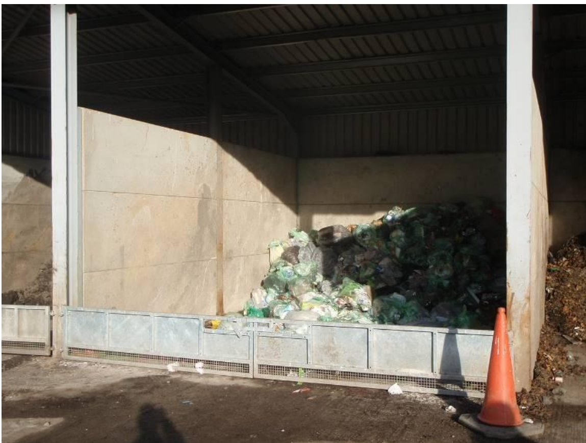
Photograph above shows bay being used for collected parks and garden waste
