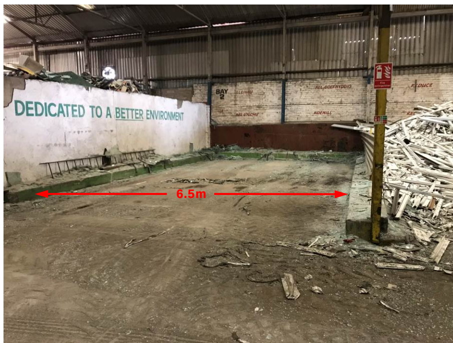
Glass Storage Bunker
